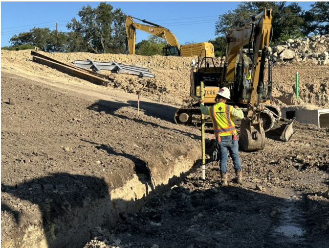
Trench for Toe Drain
