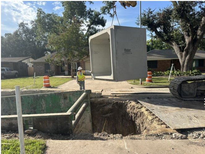
Storm Sewer Installation
