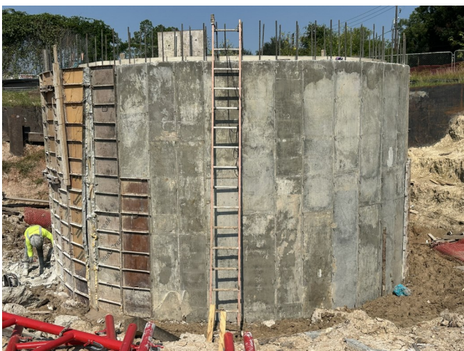
Wet Well Concrete
