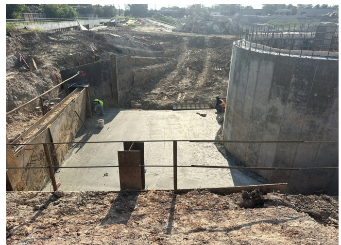
Valve Vault Concrete
