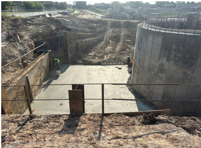
Valve Vault Concrete
