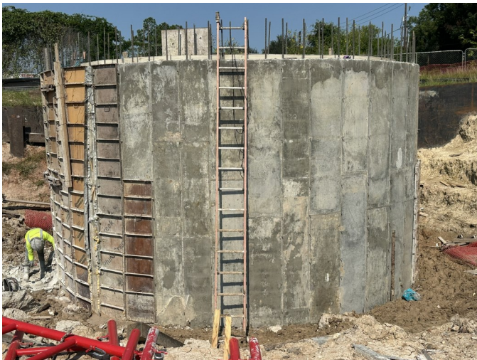
Wet Well Concrete
