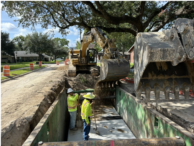
Storm Sewer Installation on Windhover
