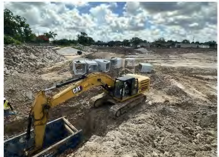
Storm Sewer Trench Excavation
