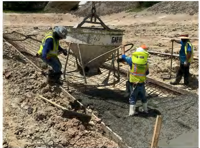
Concrete Pilot Channel
