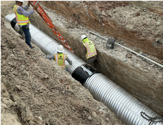
Storm Sewer Installation
