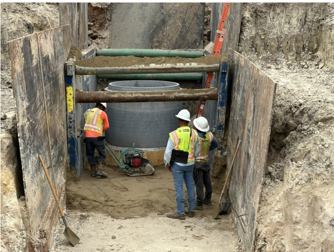
Manhole Installation
