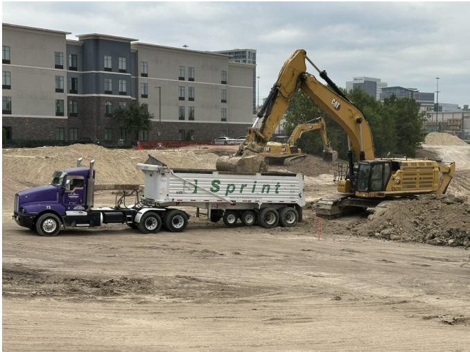
Excavation and Offsite Disposal
