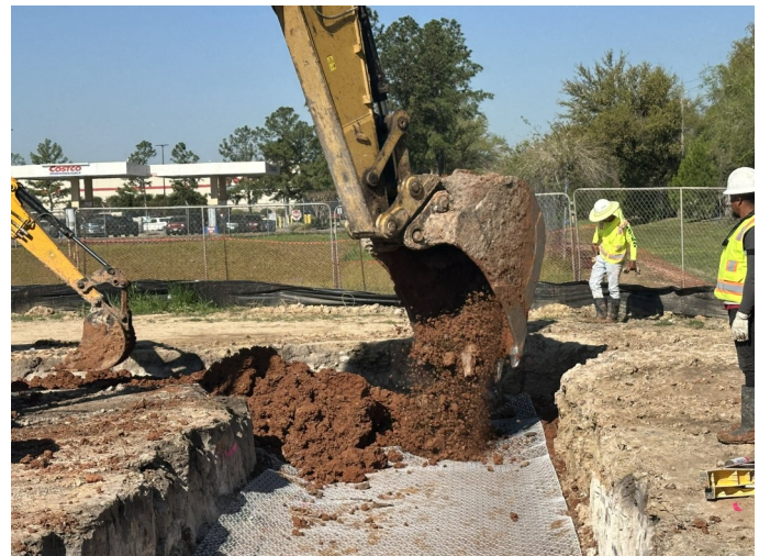
Geogrid and Clay Cap Installation
