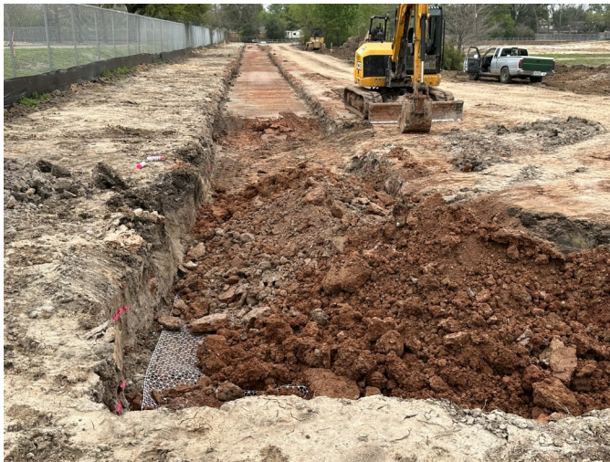
Slurry Wall Clay Cap Installation
