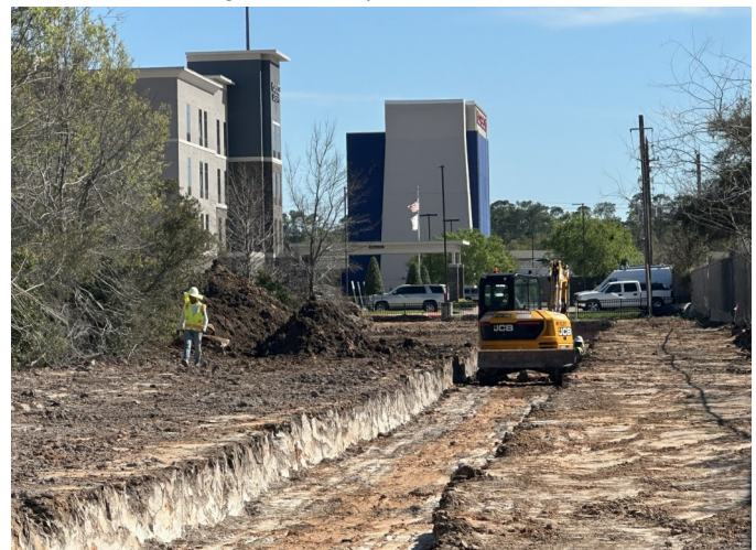
Slurry Wall Clay Cap Compaction
