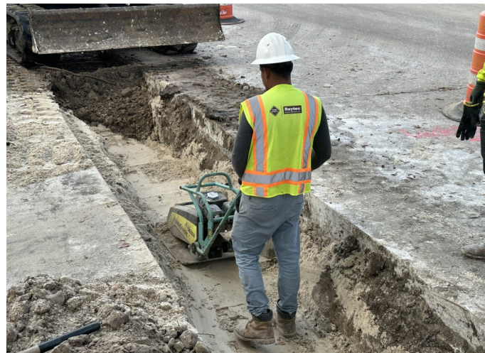
Backfill and Compaction
