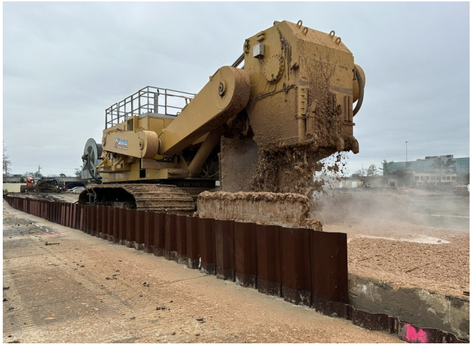
Slurry Wall Installation
