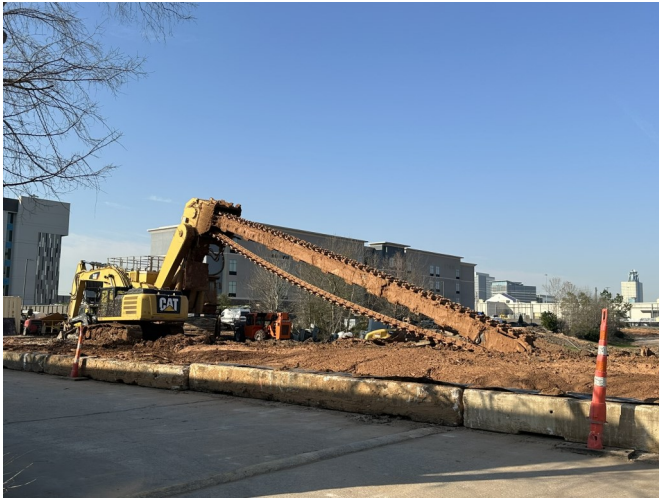
Slurry Wall Equipment
