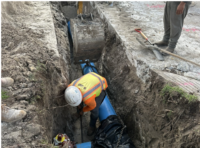
Water Line Installation
