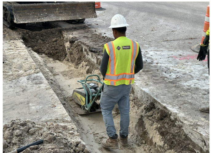
Backfill and Compaction
