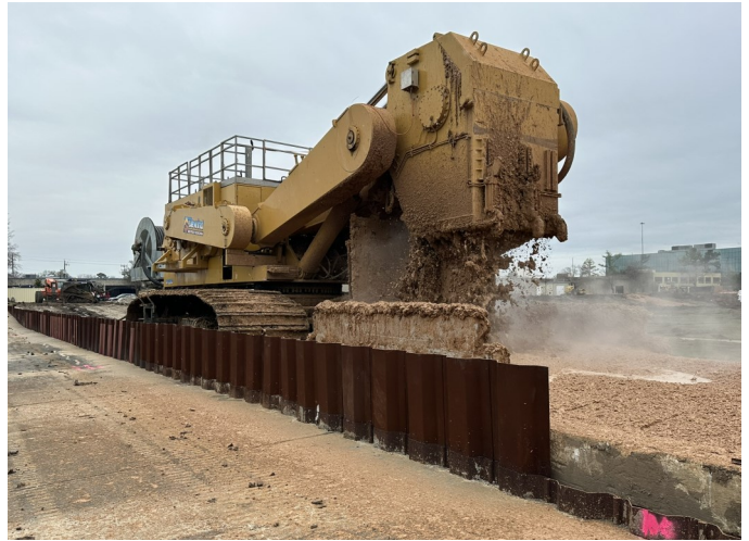
Slurry Wall Installation
