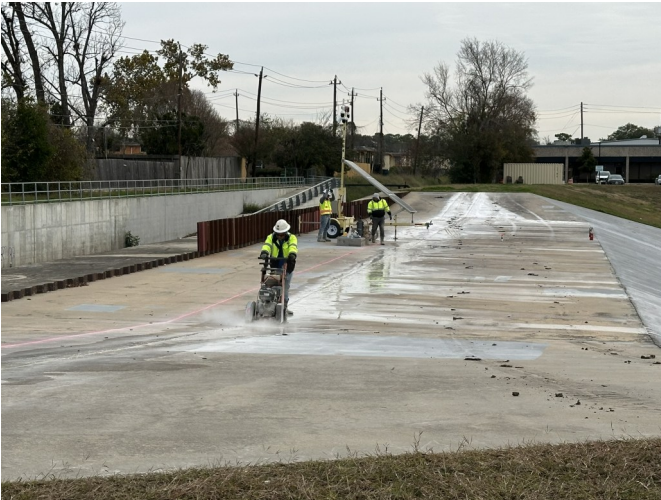
Saw cut weir for subsurface barrier wall
