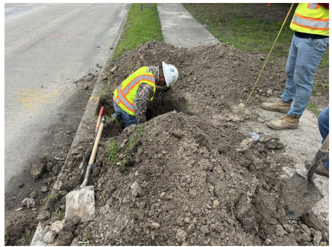
Locating existing utilities
