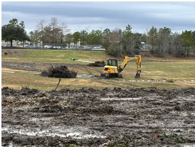
Clearing and grubbing
