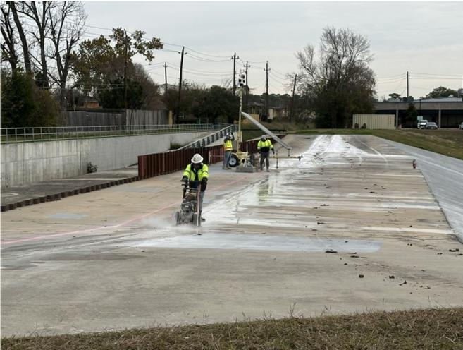
Saw cut weir for subsurface barrier wall
