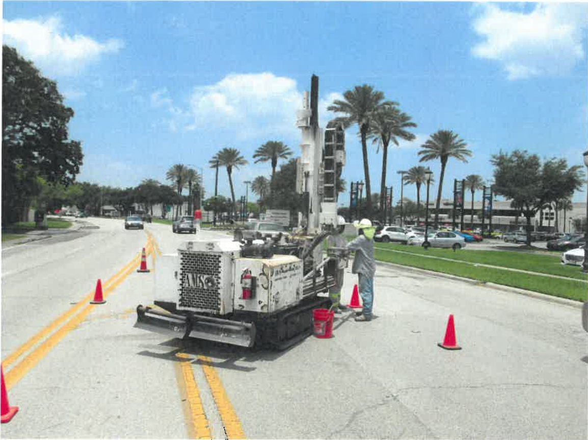
Photograph 1: View to the northwest of the drilling of soil boring B-11 on Memorial Drive in PPCAs #2, 3, and 4.
