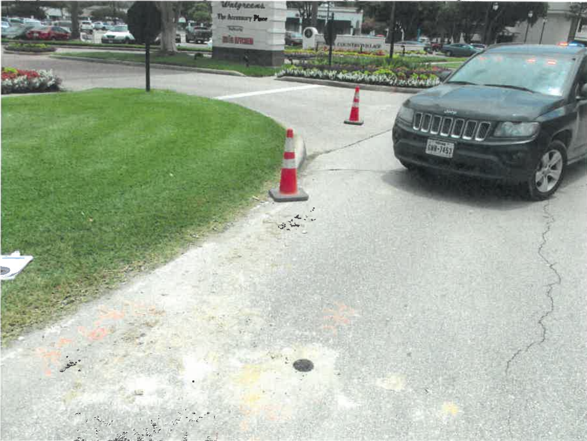
Photograph 12: View of pavement patch at soil boring B-9.
