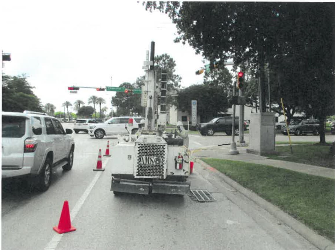
Photograph 2: View to the north-northwest of the drilling of soil boring B-15 on Memorial Drive in PPCAs #2, 3, and 4. The source of the dry cleaner leak is right of photograph down West Bough Lane (cross street in photograph) A former leaking gasoline station was located at the current Chase Bank.
