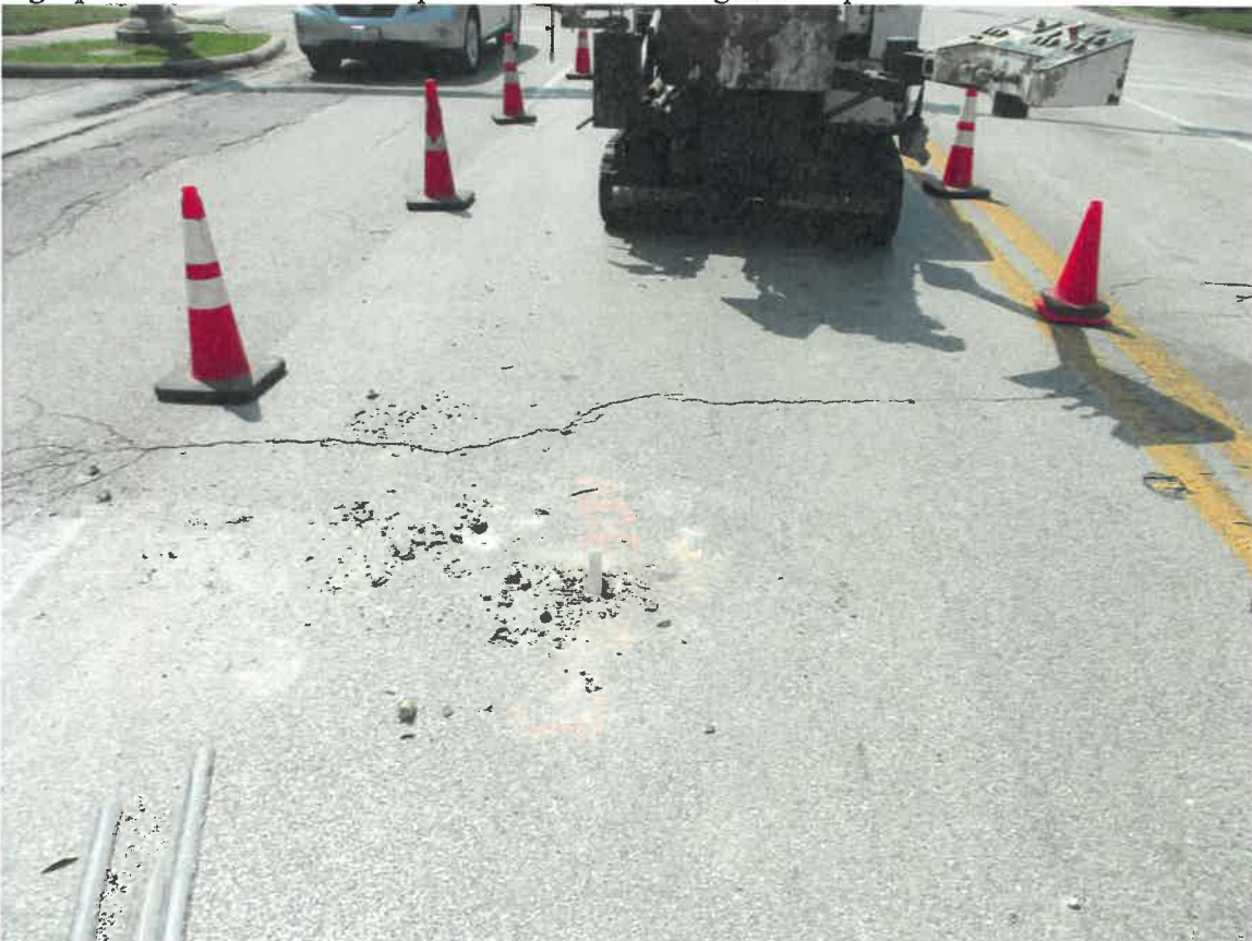
Photograph 10: View to the southeast of the temporary monitoring well installed at the B-13 boring location.
