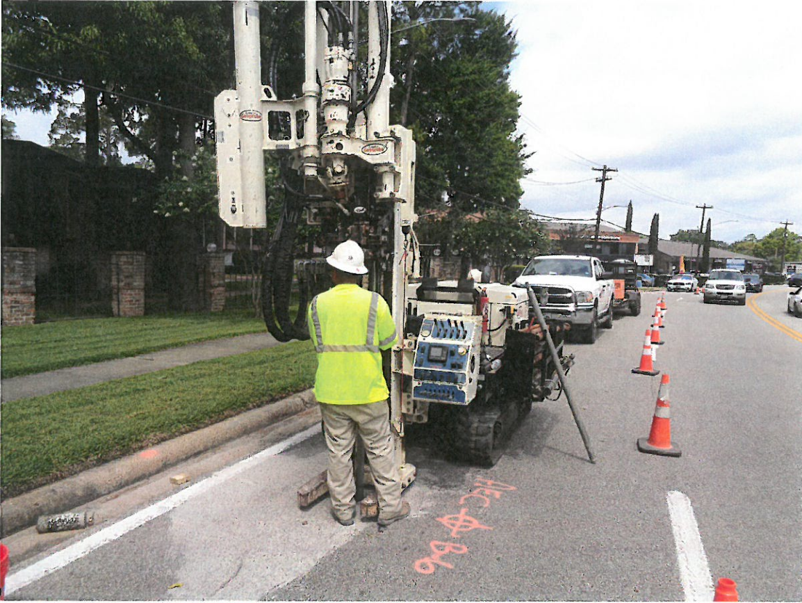
Photograph 5: View to the west of the drilling of soil boring B-6.
