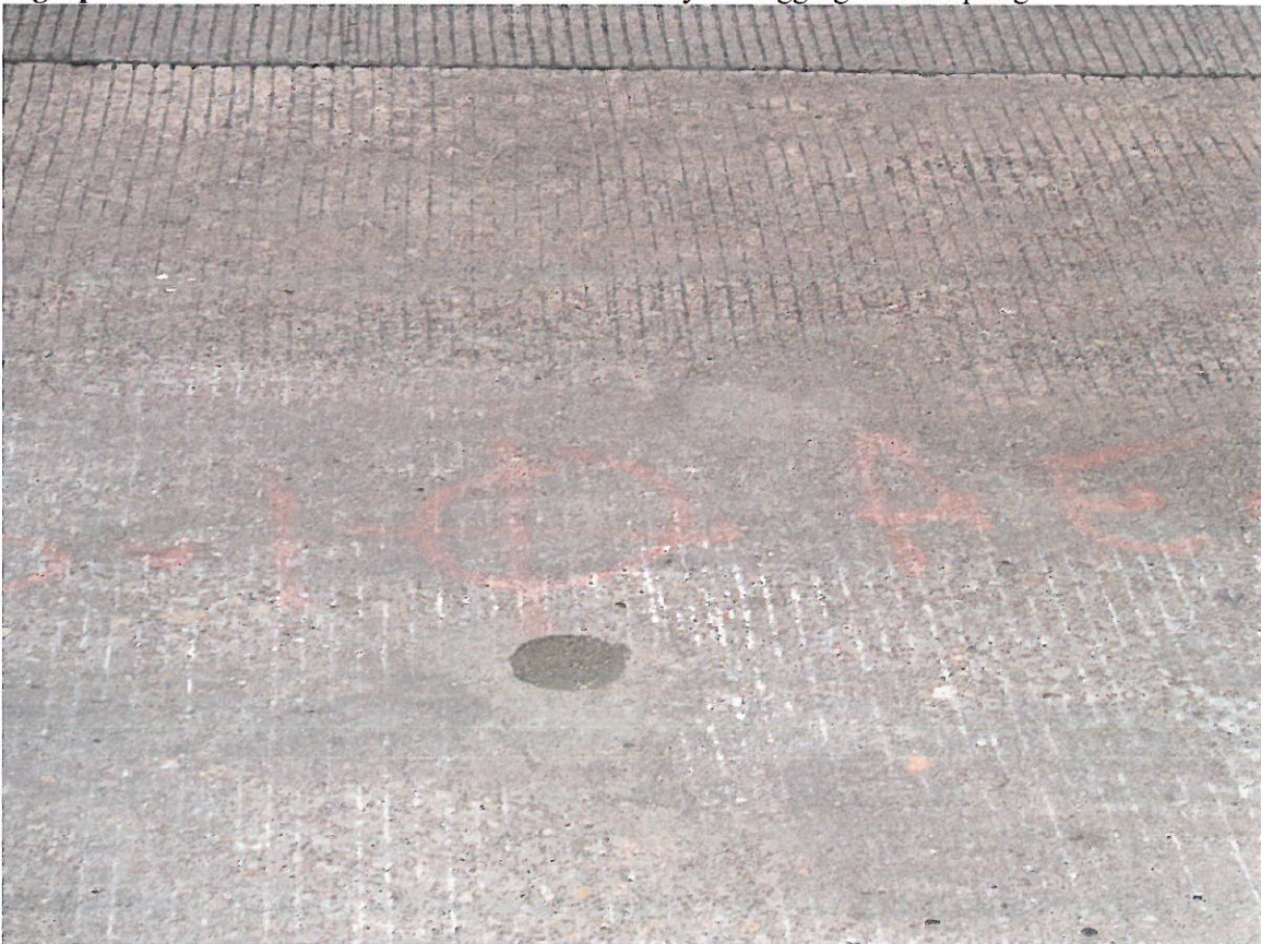
Photograph 8: View to the west of plugged and patched boring B-1.
