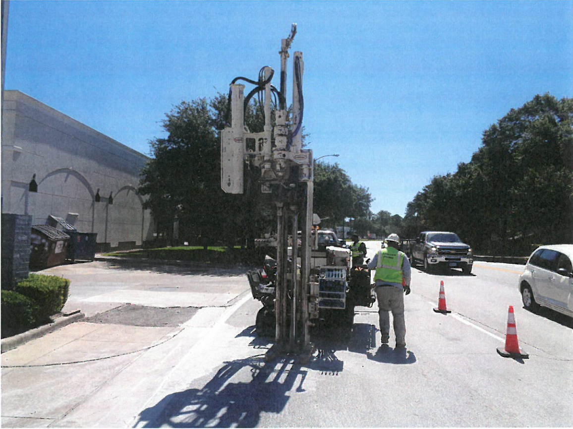
Photograph 3: View to the west of the drilling of soil boring B-3.
