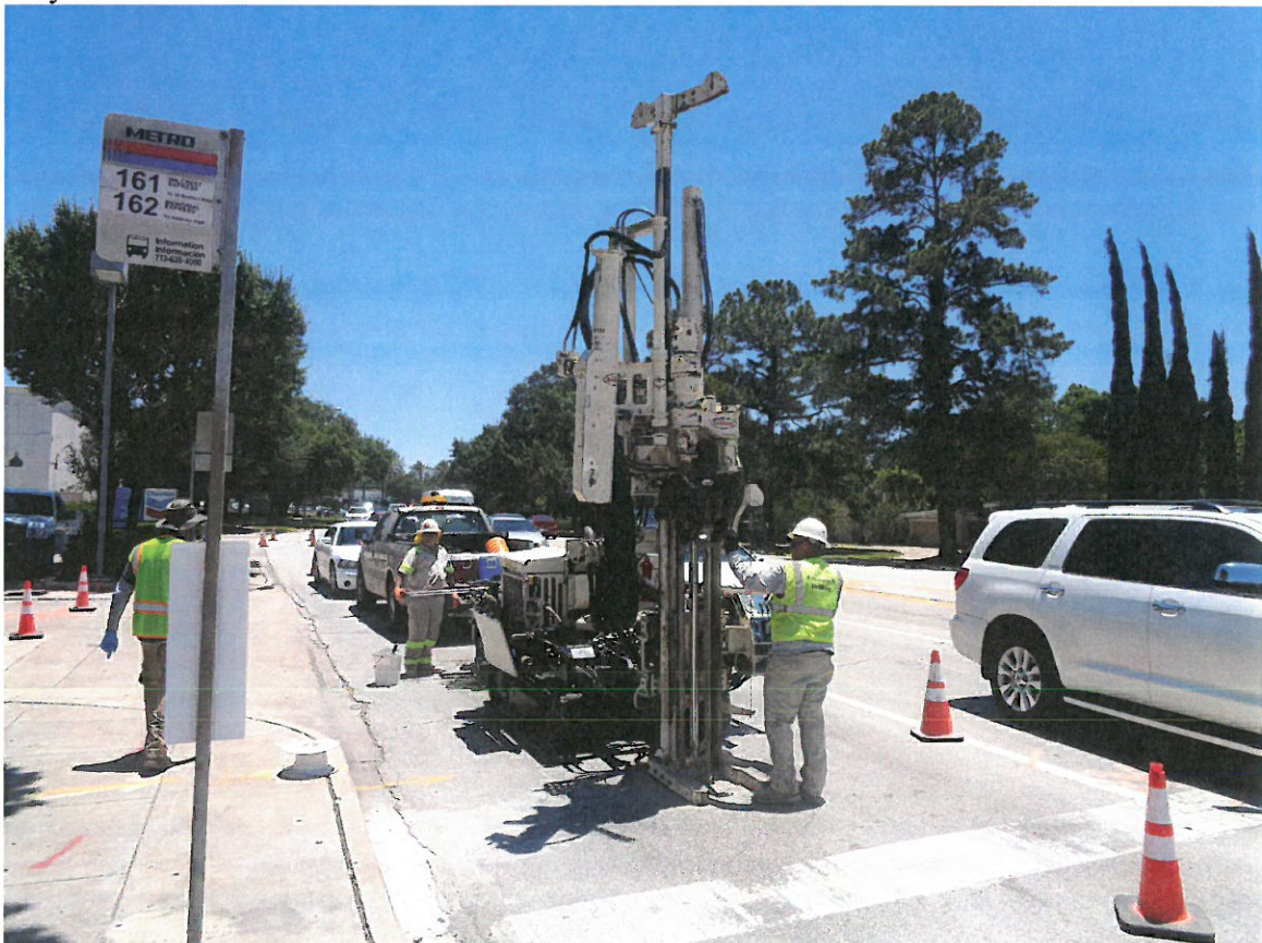
Photograph 2: View to the west of the drilling of soil boring B-2.
