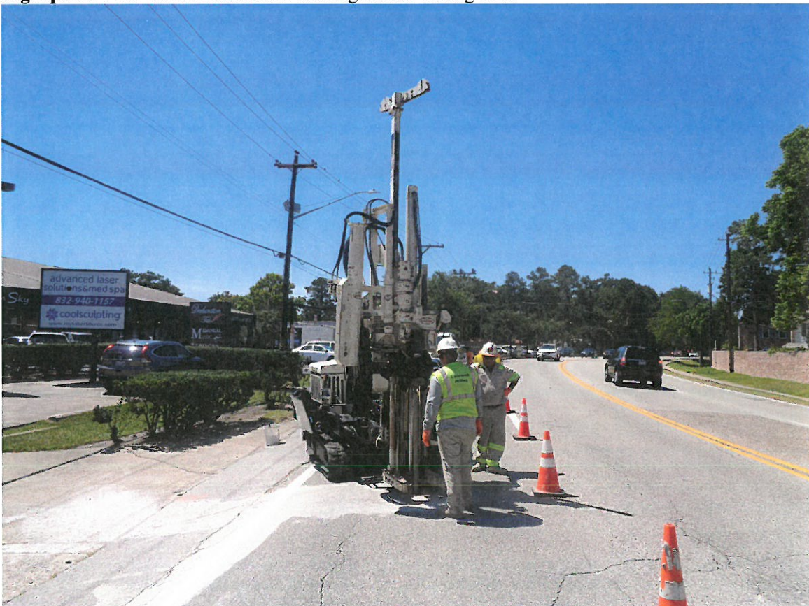
Photograph 4: View to the north of the drilling of soil boring B-4.
