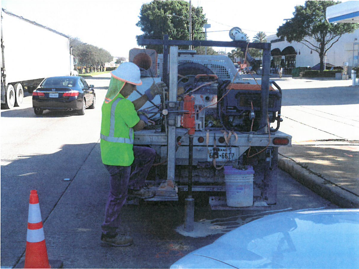
Photograph 1: View to the north of the pavement coring of location B-1 on the West Sam Houston Parkway South.
