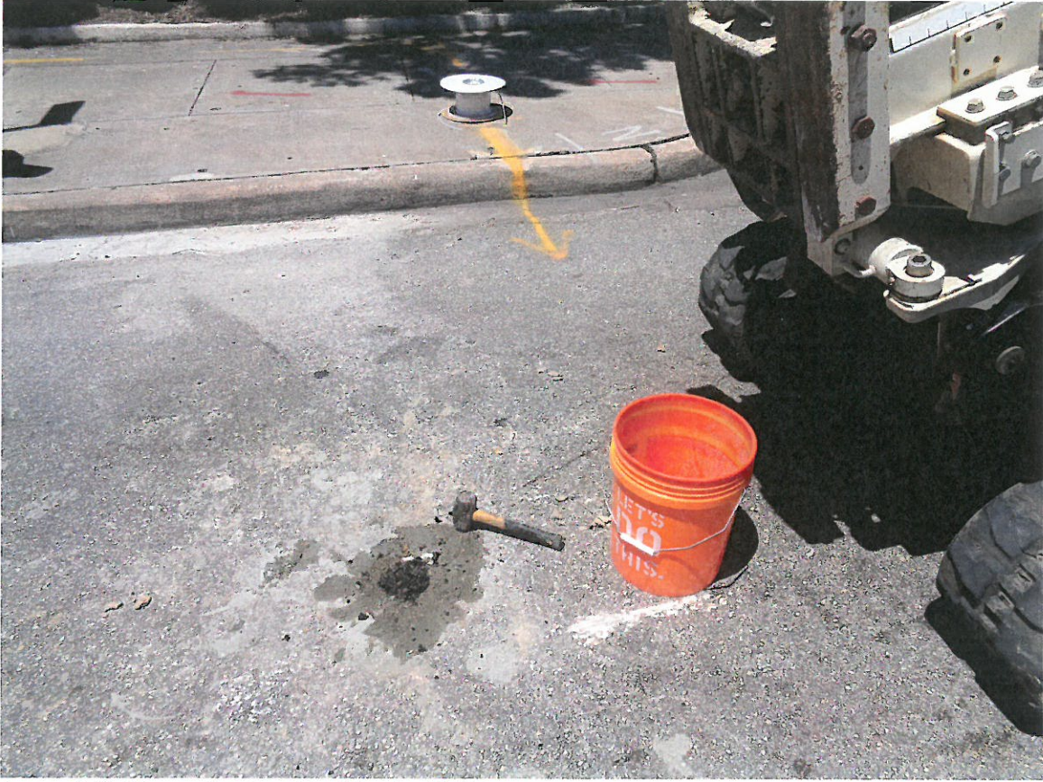
Photograph 9: Plugged and patched boring B-2.
