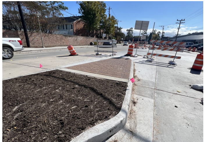
Median Installation Completed
