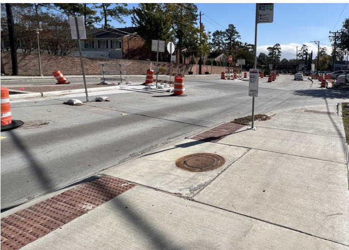
Completed Sidewalk & Bus Stop
