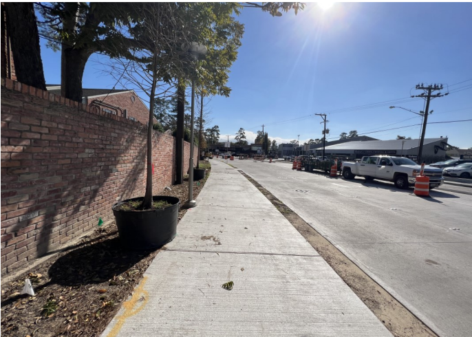
Landscaping in Progress
