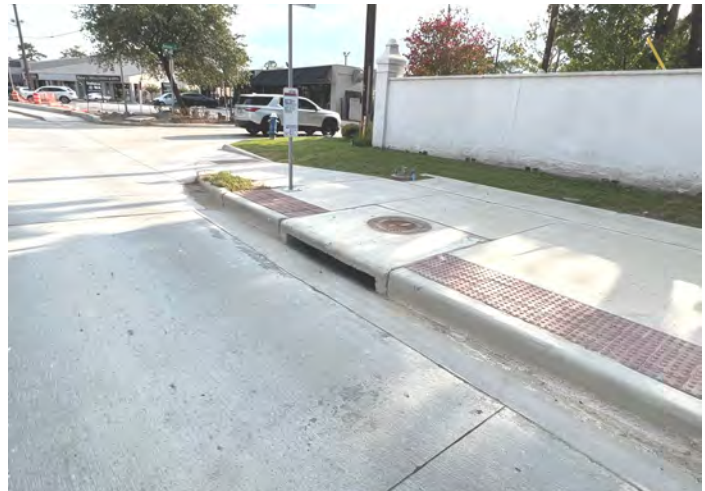
Completed Inlet Installation
