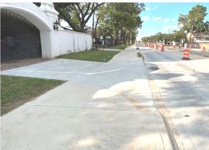
Completed Sidewalk and Driveway
