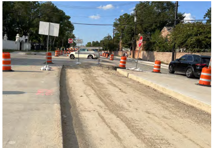
Raised Median Installation
