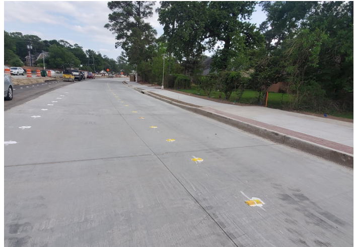
New Concrete Pavement
