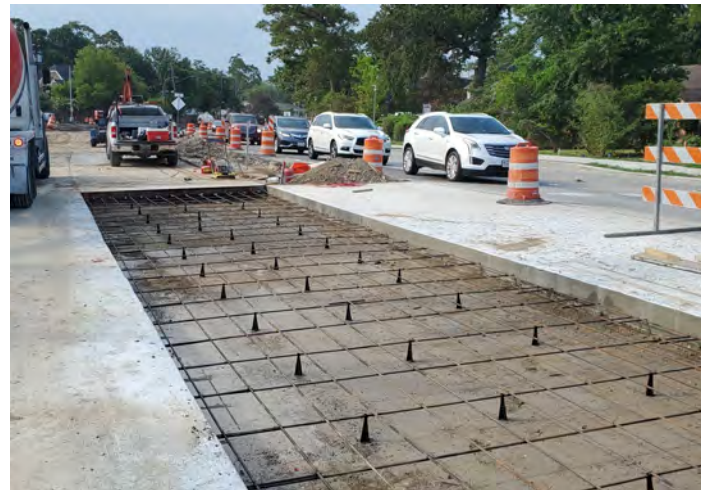
Rebar Framework Installation
