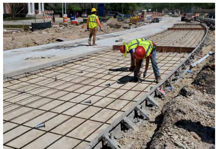
Concrete framework installation in progress
