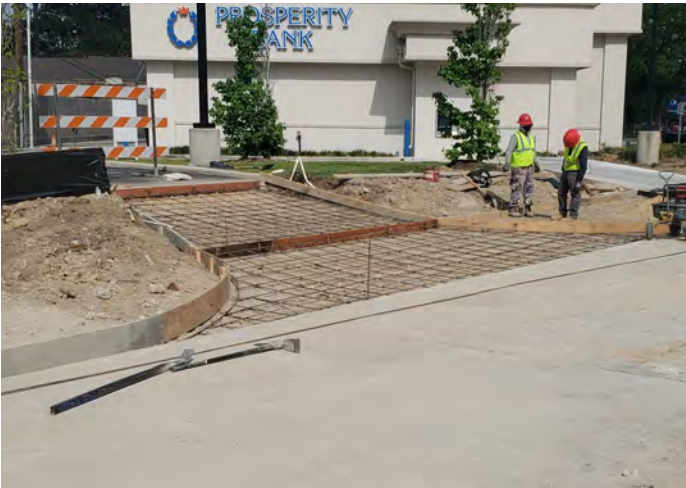
Driveway framework installation in progress
