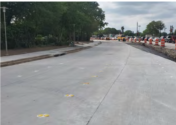
New concrete pavement
