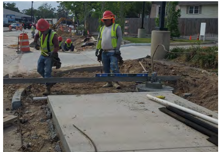
Sidewalk installation in progress
