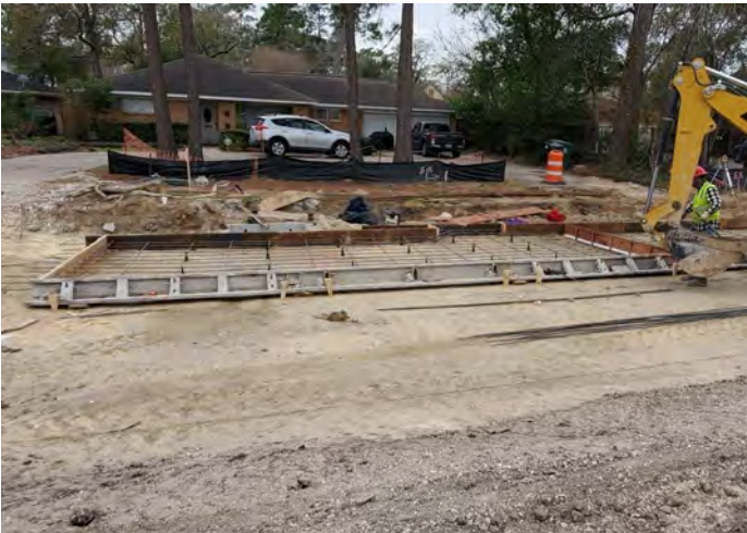
Roadway framework installation in progress
