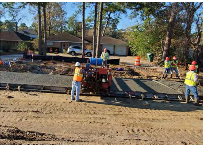
Concrete roadway installation in progress
