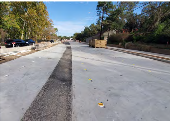
Roadway construction in progress
