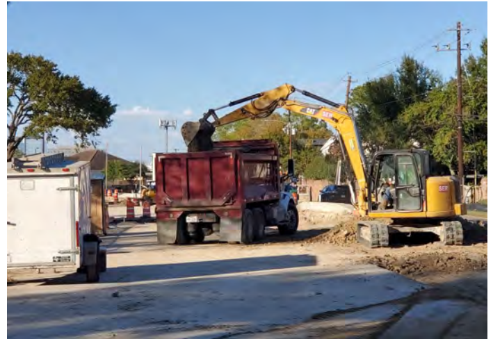
Roadway Excavation in progress
