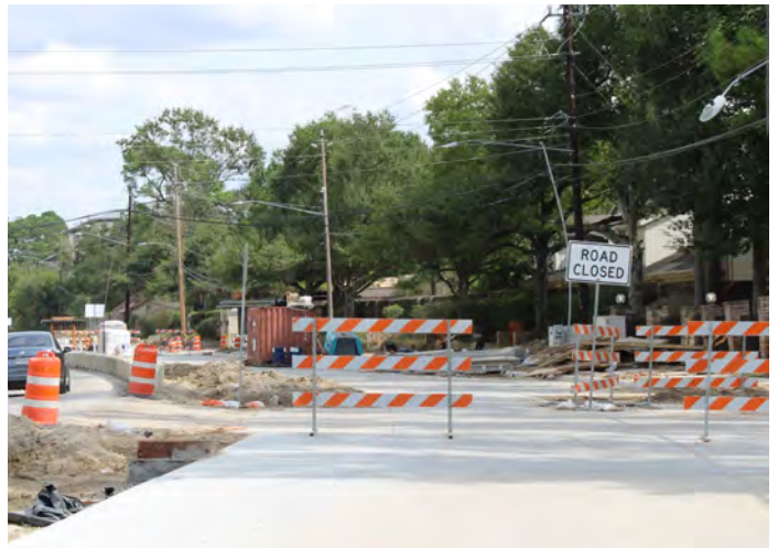
Traffic Control setup
