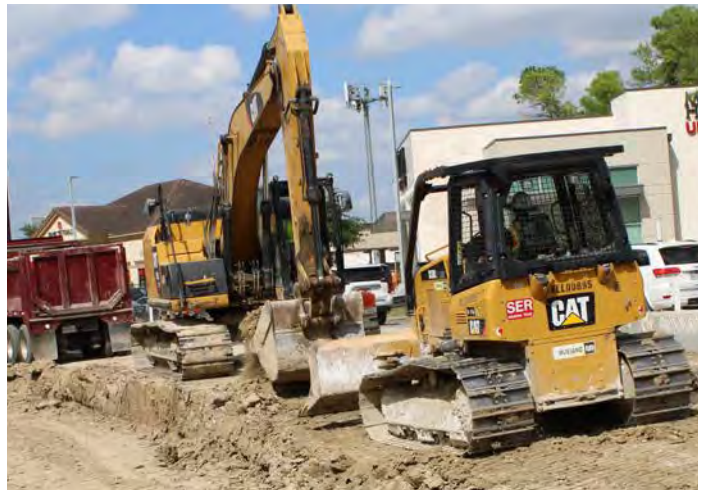
Roadway Excavation in progress
