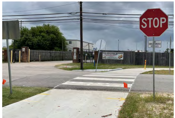
Crosswalk Completion - Witte Road
