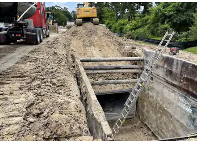
10-ft x 5-ft Storm Sewer RCB Installation
