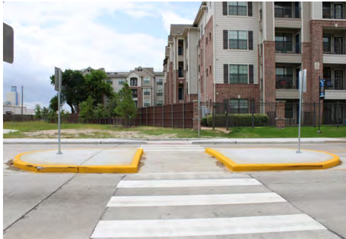
Crosswalk Island Completion - Bunker Hill Rd
