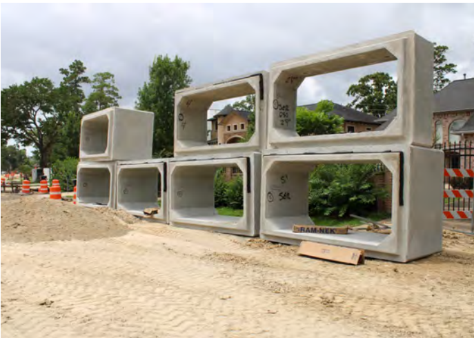
10-ft x 5-ft Storm Sewer RCB Stockpile
