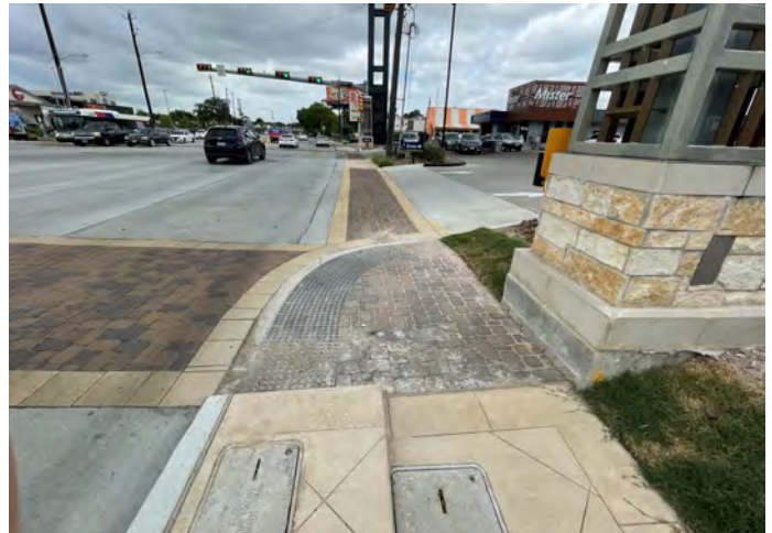
Intersection Curb Ramps at Mathewson — Completed
