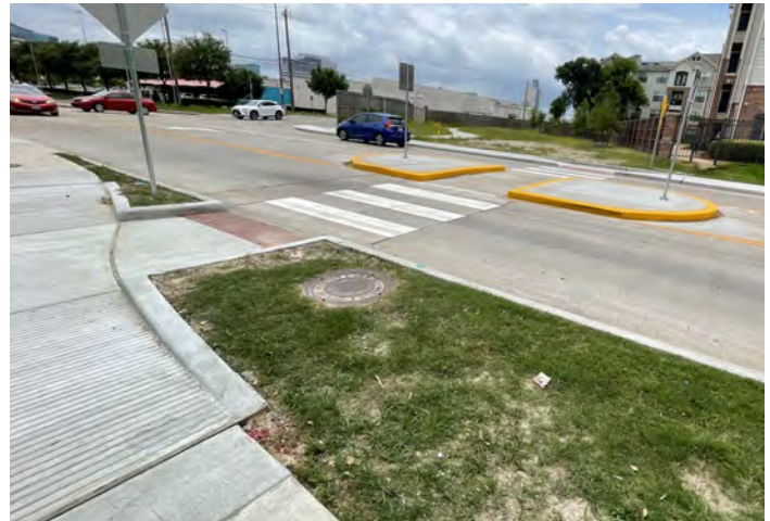
Crosswalk Completion - Bunker Hill Rd
