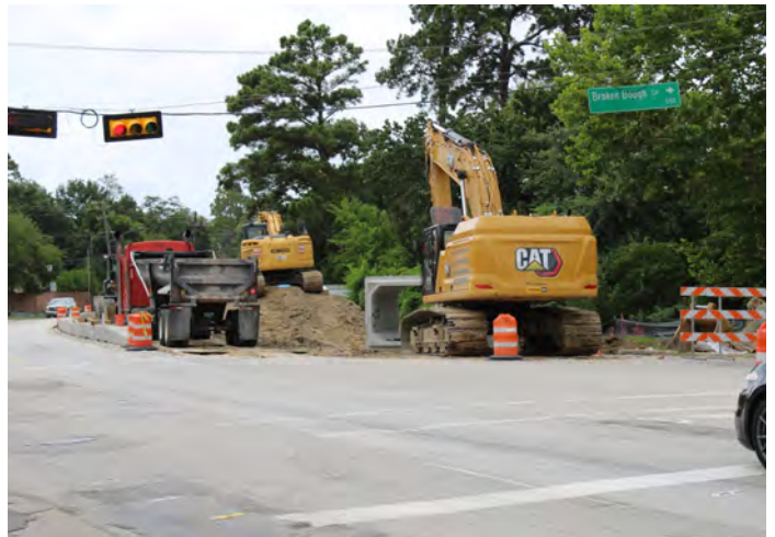
10-ft x 5-ft Storm Sewer RCB Installation
