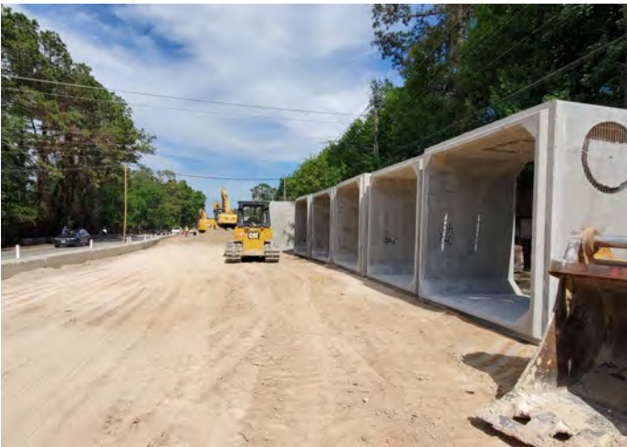
10-ft x 10-ft Storm Sewer RCB Stockpile
