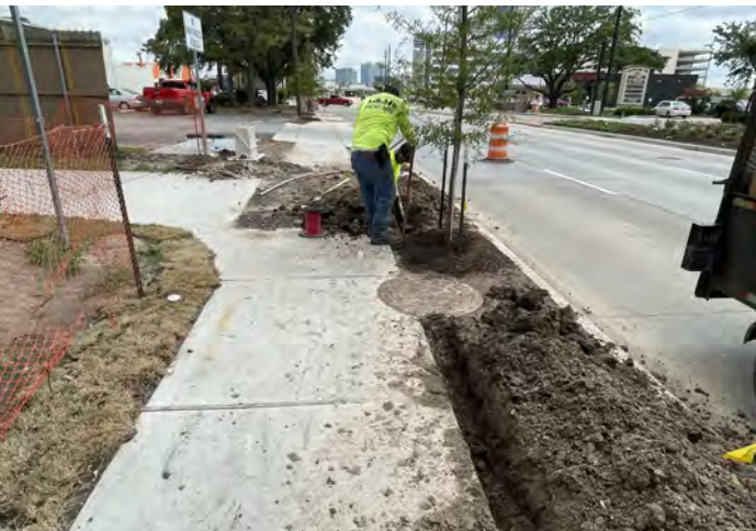
Landscaping Work—Almost Completed
