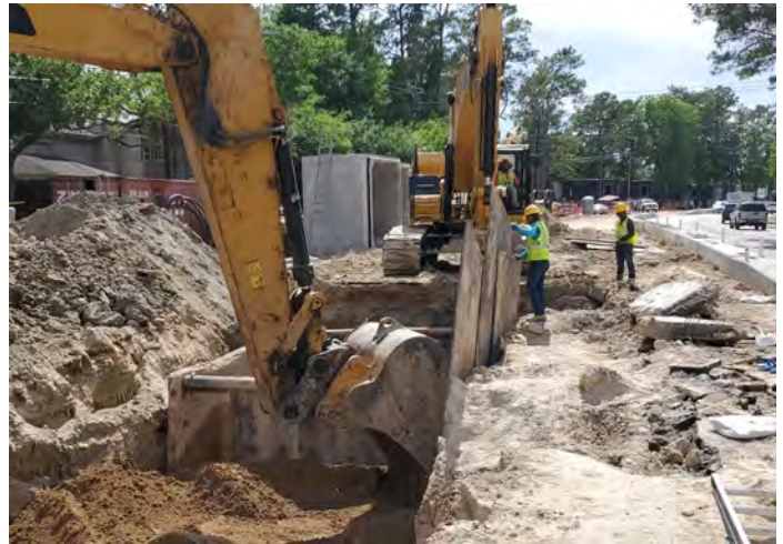
10-ft x 10-ft Storm Sewer RCB Installation
