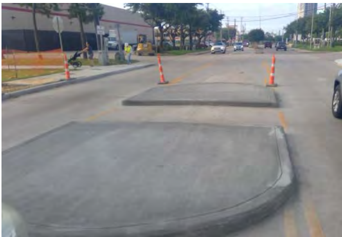
Crosswalk Island Completion - Bunker Hill Rd
