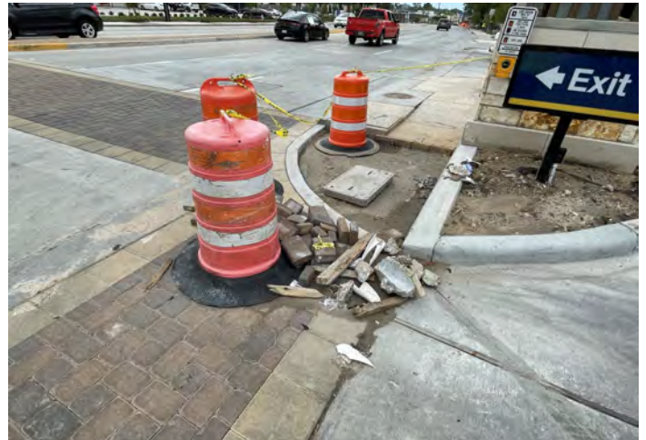
Intersection Curb Ramps at Mathewson—In progress
