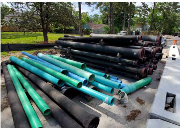
Water line & Sanitary line Stockpile
