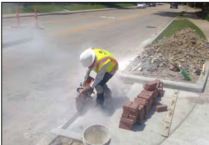
Truncated Domes Installation - Bunker Hill Rd
