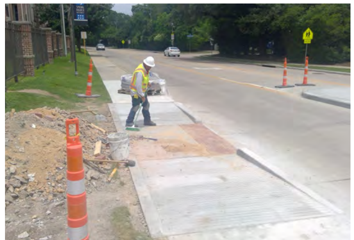
Ramp Work Completed—Bunker Hill Rd
