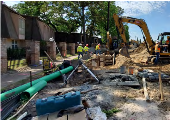
Water Line Installation work
