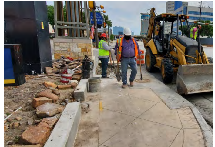
Back of Curb Improvements —In progress
