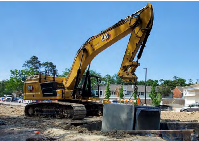
10-ft x 10-ft Storm Sewer RCB Installation
