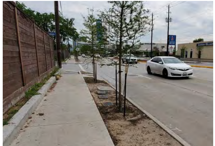
Landscaping Work—In progress
