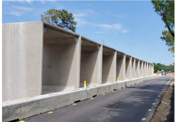
10-ft x 10-ft Storm Sewer RCB Stockpile
