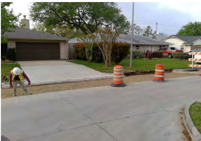
Replaced pavement—Long Branch
