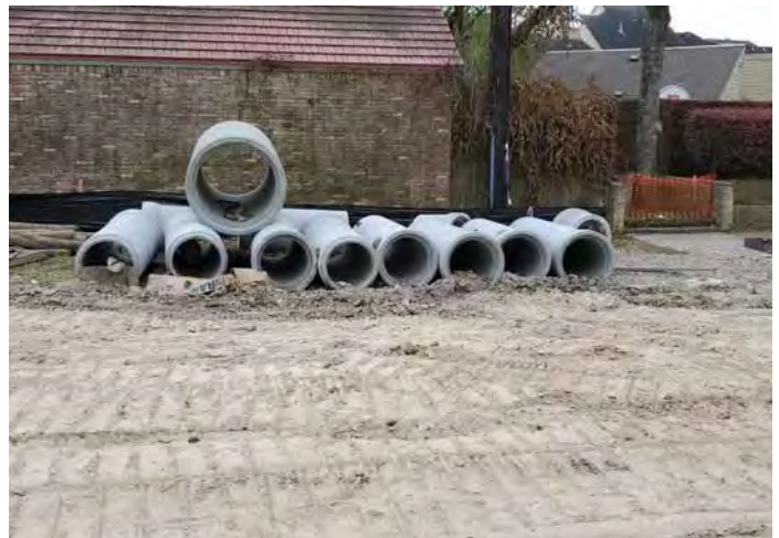
Storm Sewer RCP Stockpile
