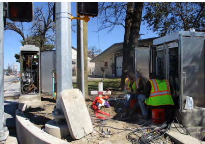
Wiring Traffic Signal Controllers at Westview Drive
