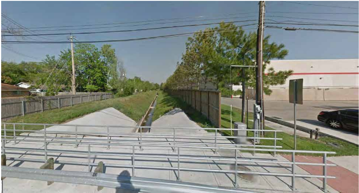
Pre-construction: On Bunker Hill looking east.
