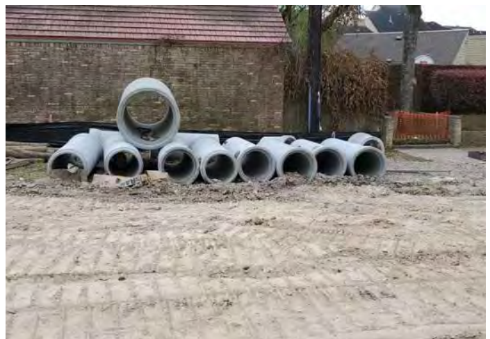
Storm Sewer RCP Stockpile
