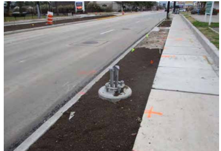
Street Light Foundations—In progress
