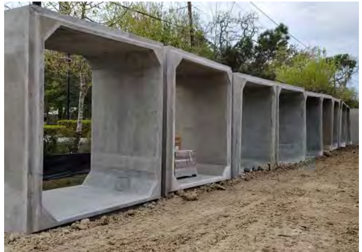
10-ft x 10-ft Storm Sewer RCB Stockpile
