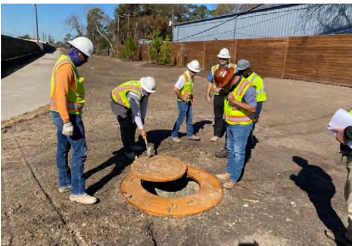
Substantial Completion Walkthrough with City staff
