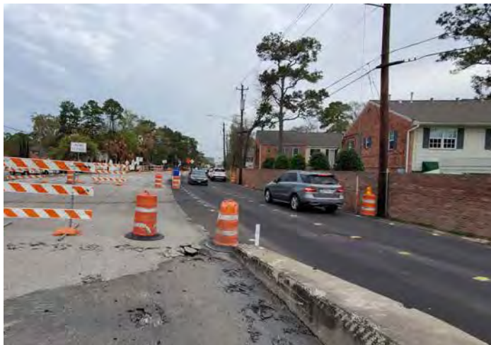
Current Traffic Control Configuration
