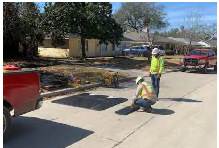
Installing road cushions on Long Branch
