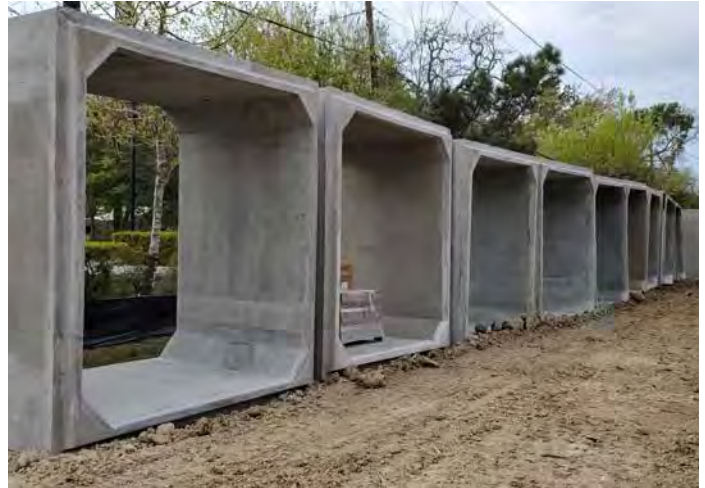
10-ft x 10-ft Storm Sewer RCB Stockpile
