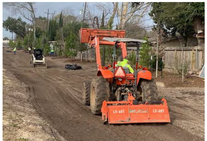
Spreading top soil
