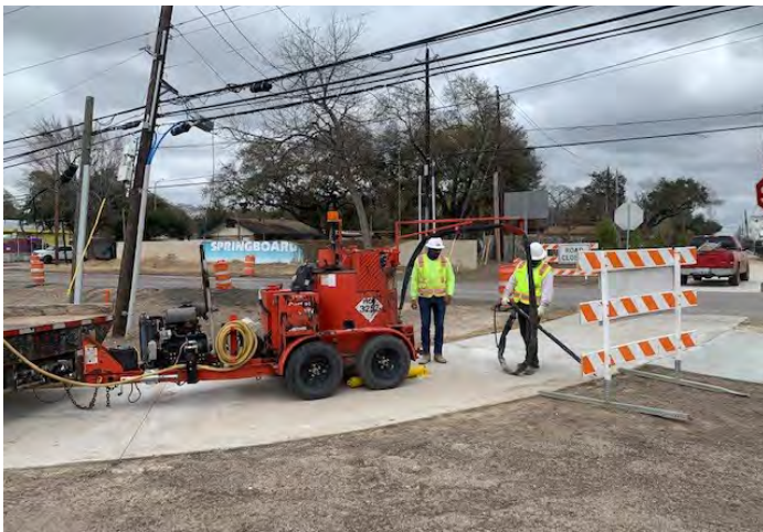
Applying sealant to Access Road
