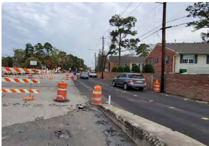
Current Traffic Control Configuration
