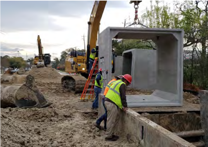
10-ft x 10-ft Storm Sewer RCB installation at W153
