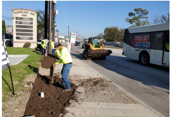
Landscaping and Irrigation Meters Installation in progress
