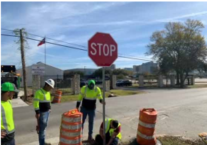
Signs Installation at Witte Rd—Completed
