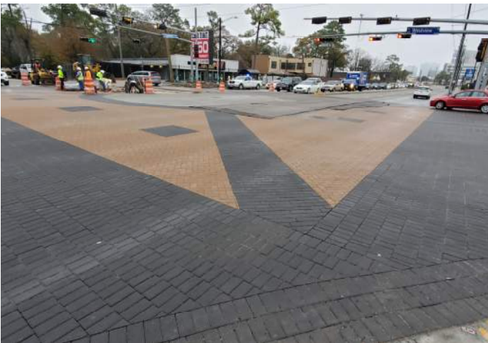
Brick Pavers Installation at Westview Intersection—Completed
