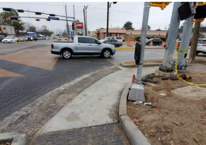
Truncated Domes at Westview Intersection—Completed
