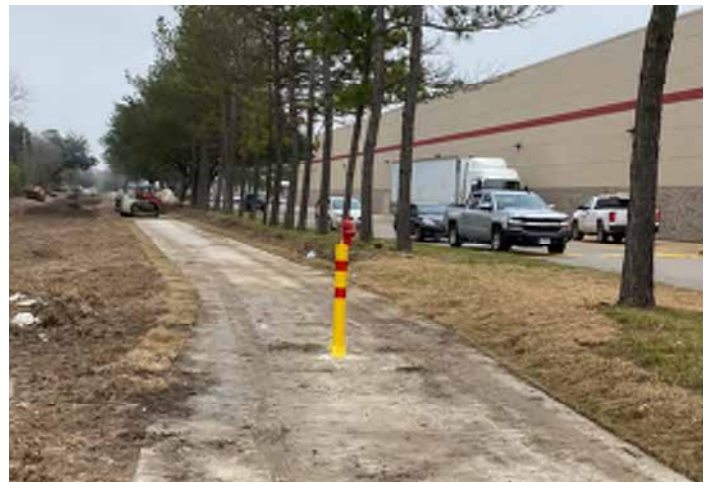
Bollards Installation —Completed
