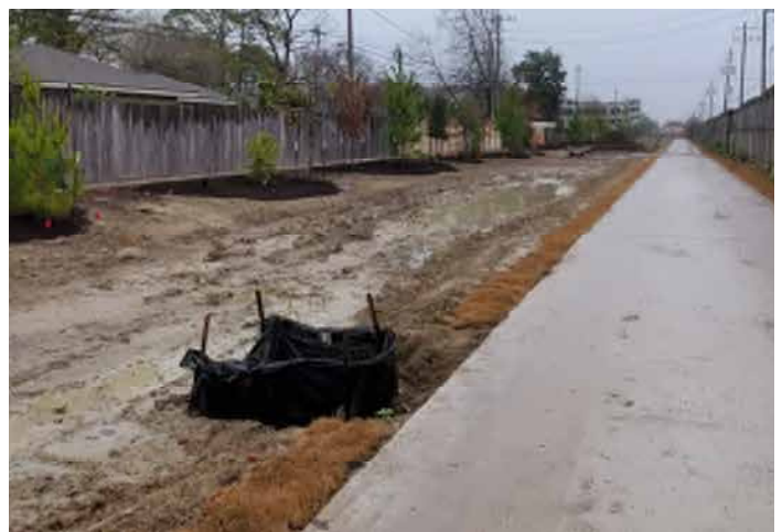
Erosion Control & Soil Remediation— In Progress
