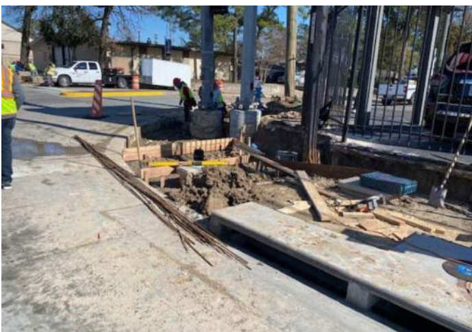
Frame Work for Sidewalk –SE corner of Westview inter section
