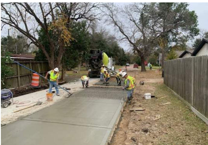
Repairing Concrete Pavement at Confederate Rd
