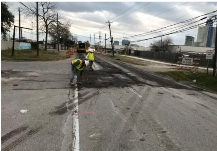
Mill and Overlay Work at Witte Rd
