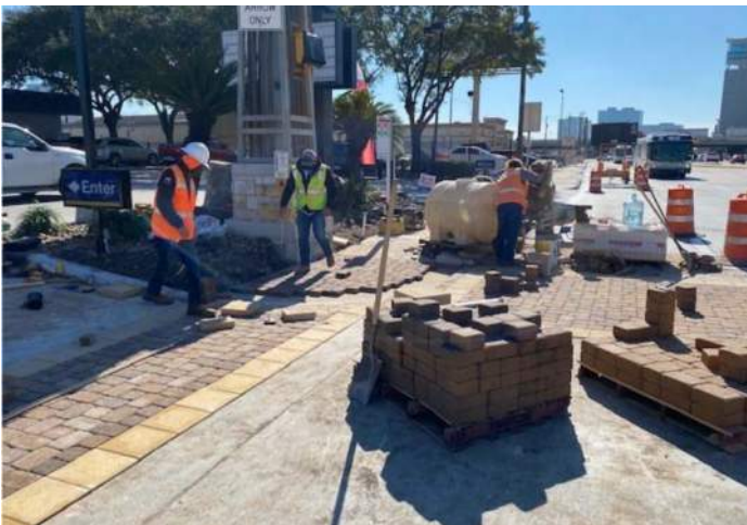
Brick Pavers Installation
