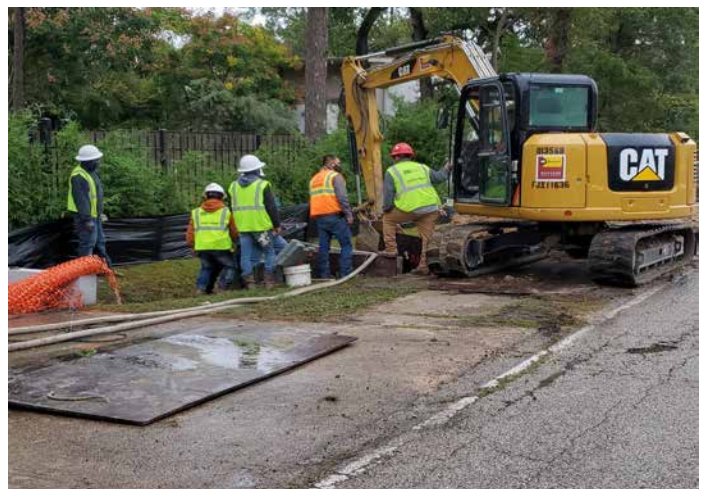
Water Line Pipe Installation
