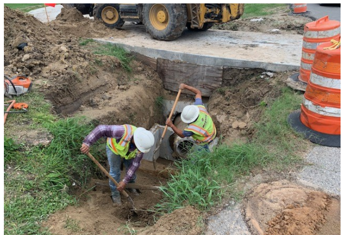
Backfilling Inlet Box at Witte Rd.
