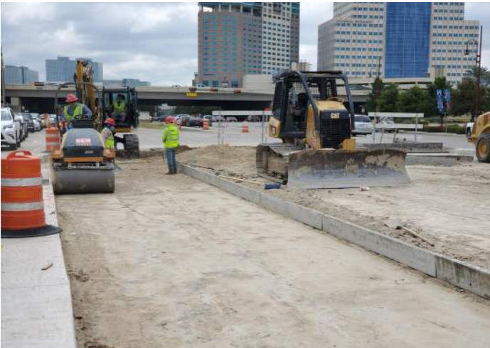
Soil compaction for travel lane - Phase 5
