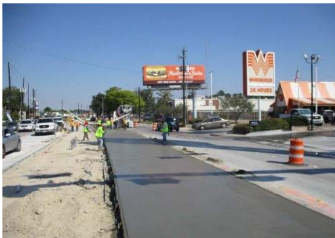
Concrete pavement for inner lanes
