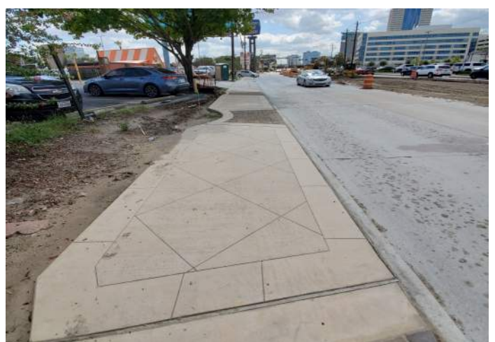
Sidewalk work ongoing on east side.
