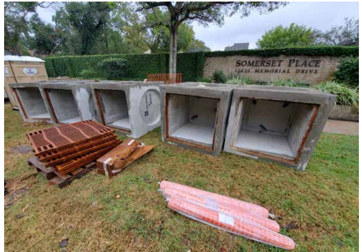
Inlets on Site
