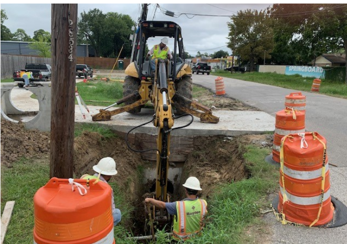
Setting Inlet on Witte Road next to Access Road.
