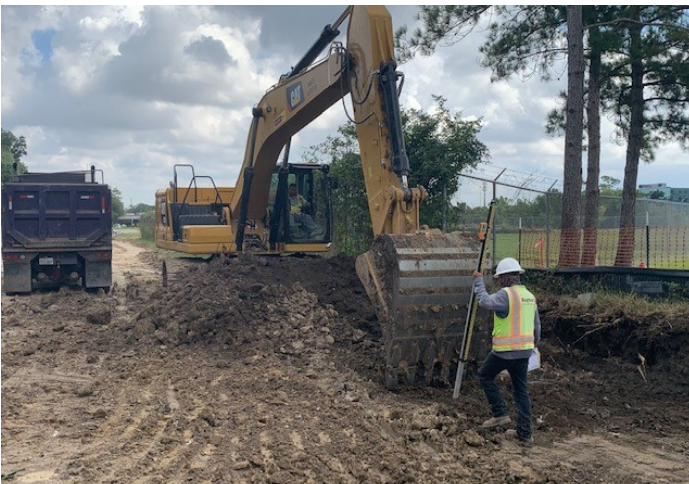
Cutting Grade for last section of Access Rd
