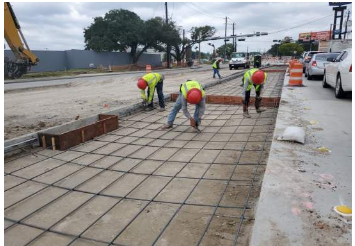
Forming work for inner travel lane (Phase 5) on east side.
