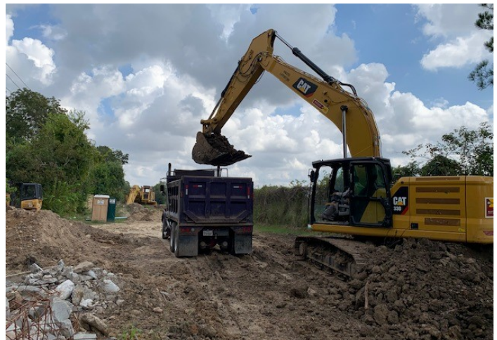
Loading Spoils into Trucks for Last Section of Access Road
