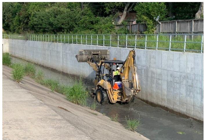
Cleaning W140 channel at the start of the project
