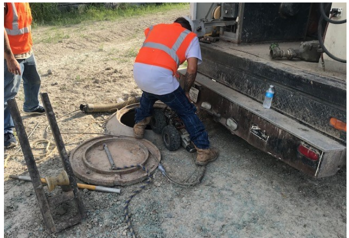
CCTV Crew Entering Storm Sewer.
