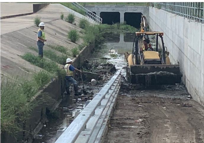
Cleaning W140 channel at the start of the project
