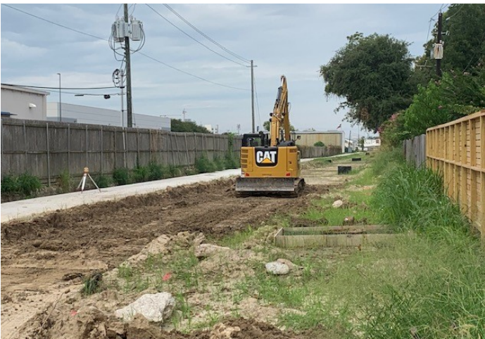
Final Grading on Phase II (Witte Road to Bunker Hill Rd)
