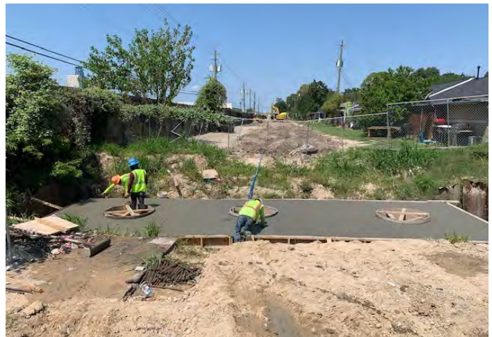
Finishing up Junction Box—Phase II.
