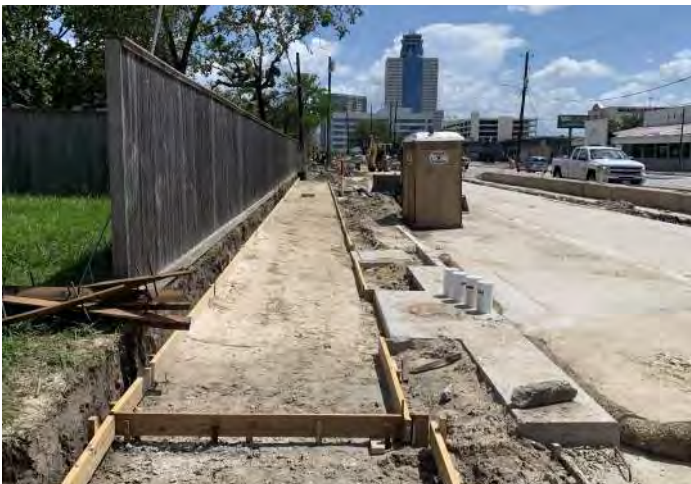
Forming work for sidewalk installation on east side.
