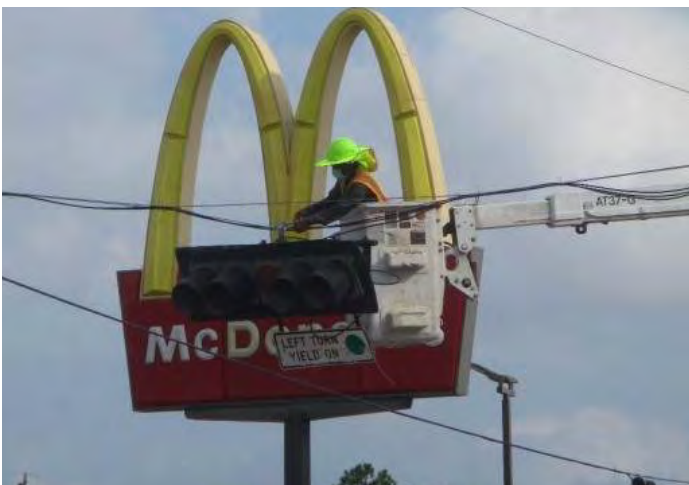
Adjusting traffic signal in preparation for traffic control changes.
