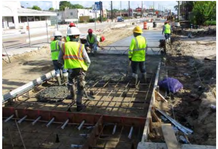
Concrete Pour on east side of Gessner Road.
