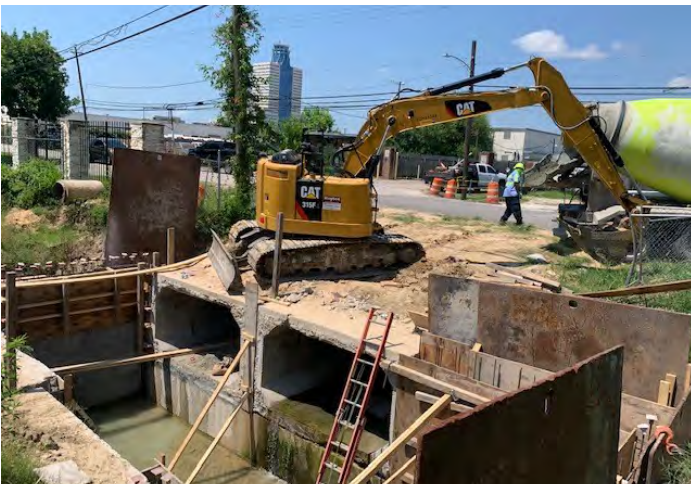
Pouring walls between the boxes at Junction Box at Witte Rd.
