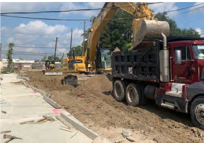
Began swale work next to Access Road
