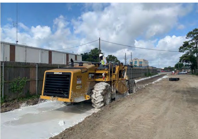
Mixing Lime Slurry (Soil Stabilization)
