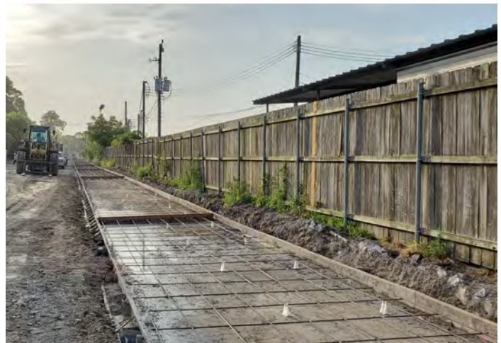
Forming of Access Road between Gessner and Witte
