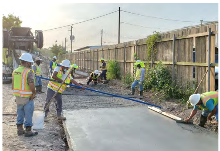
First Concrete Pour of Access Road between Gessner & Witte.
