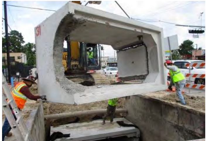
RCB installation on the east side of Gessner Rd
