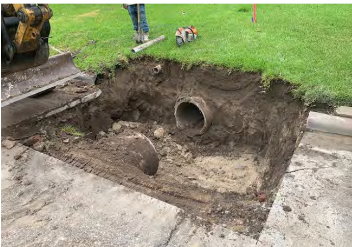
Preparing Straw 3 for inlets replacement.
