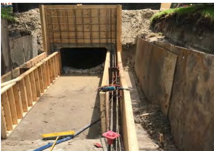
Forming wing & head walls— Long Branch & W140-01-05 (Straw 5)
