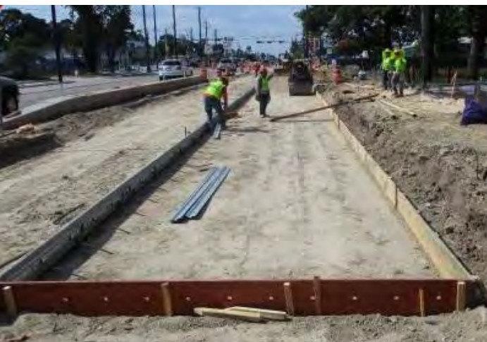
Forming work for pavement installation on east side.
