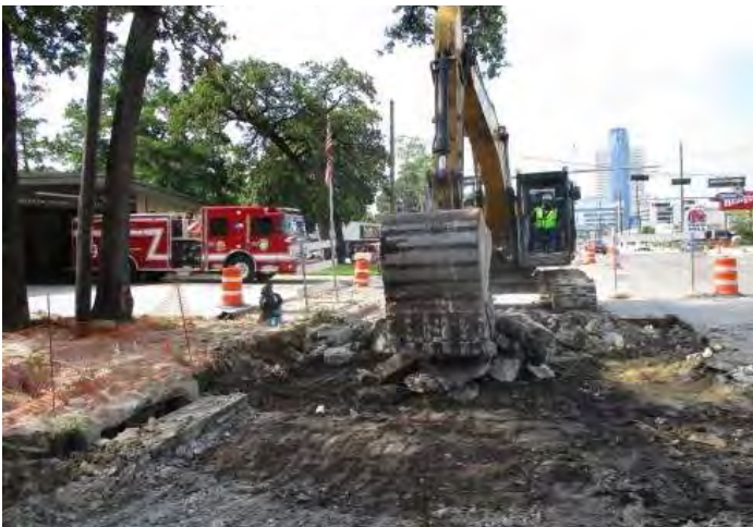
Removal of existing pavement on east side of Gessner Road
