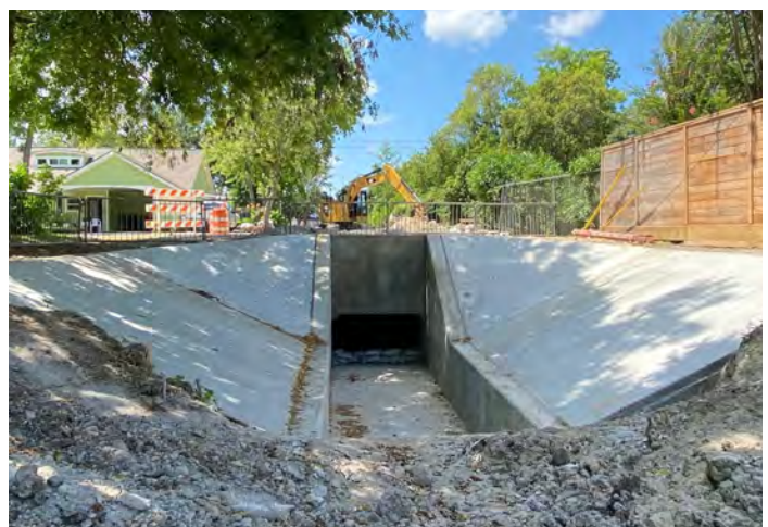
Final wing and head wall structure ( Straw 5)
