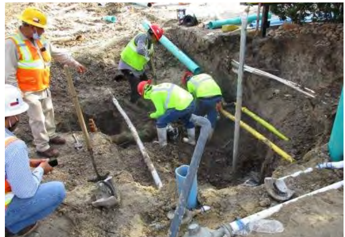
Installation of water line connections and valves
