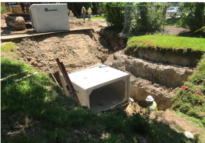
Box Installation—Long Branch & W140-01-05 (Straw 5)
