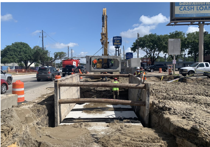
RCB installation on the east side of Gessner Rd
