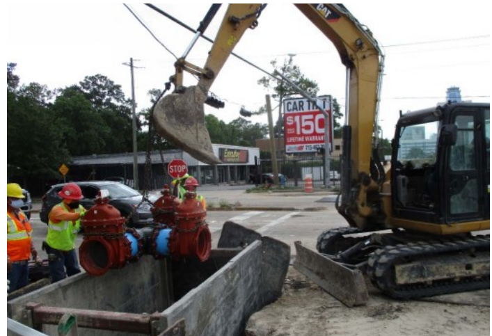
Installation of water line connections and valves
