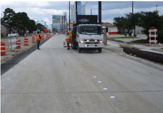
New pavement on west side of Gessner Road
