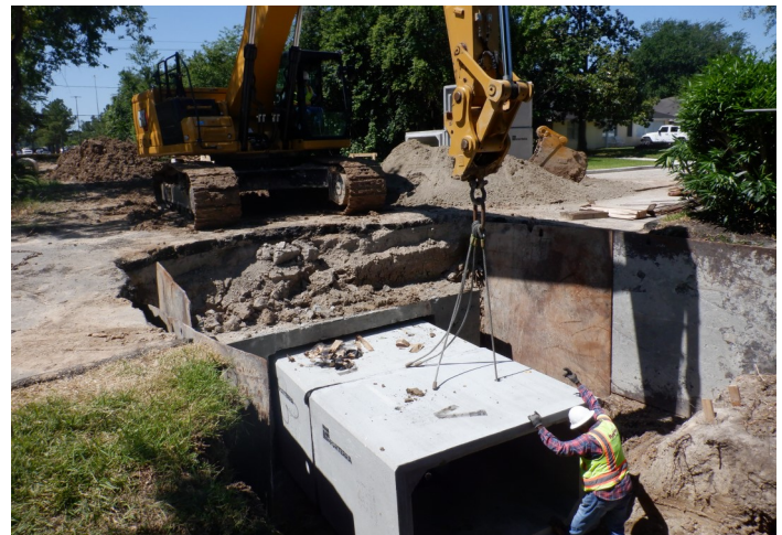
Setting RCB ( Straw 5)
