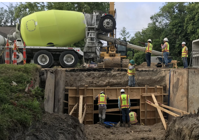
Pouring Collar— Long Branch & W140-01-05 (Straw 5)
