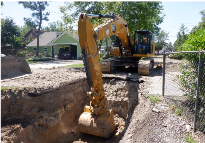
Excavation work—Long Branch & W140-01-05 (Straw 5)
