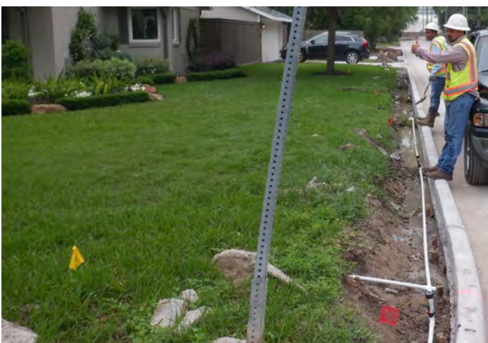
Sprinkler system repair completed Windhover Lane (Straw 4).
