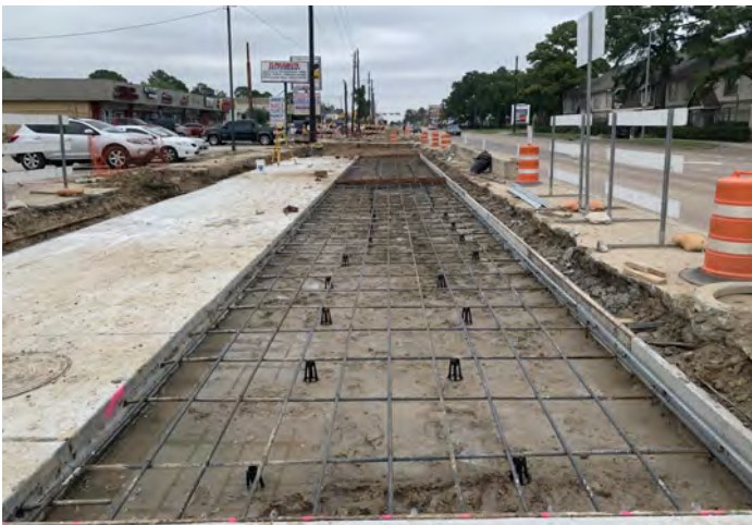
Forming and Rebar for pavement installation.
