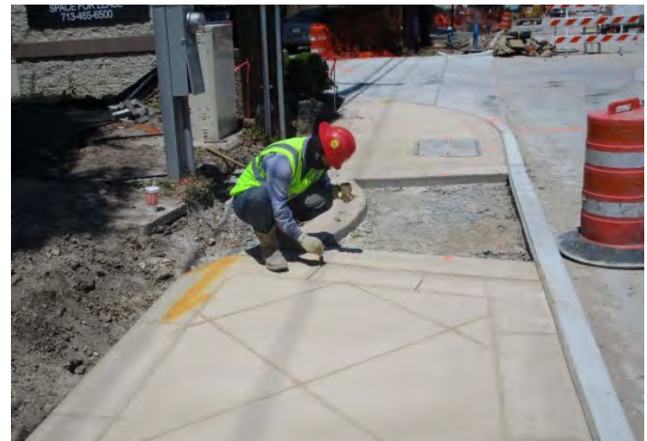
Installation of decorative sidewalks
