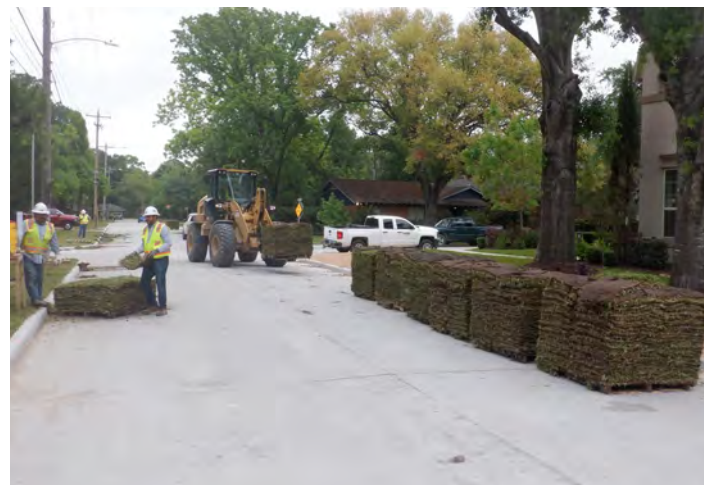
Sod installation on Windhover Lane (Straw 4)
