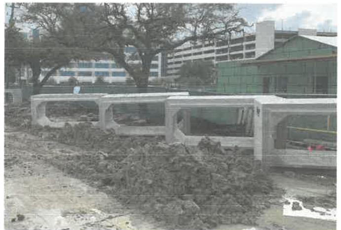
Stockpiled 10-FT x 5-FT RCBs
