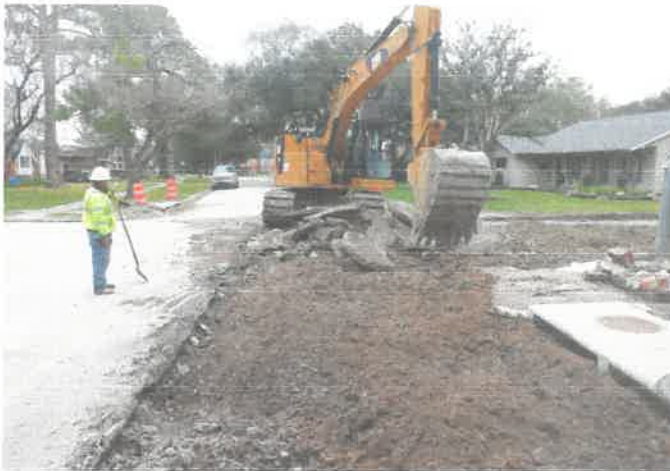
Removing Existing Paving from straw 4 to tie in connections.
