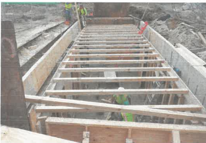
Forming junction box at intersection of straw 4 into channel (PH II)
