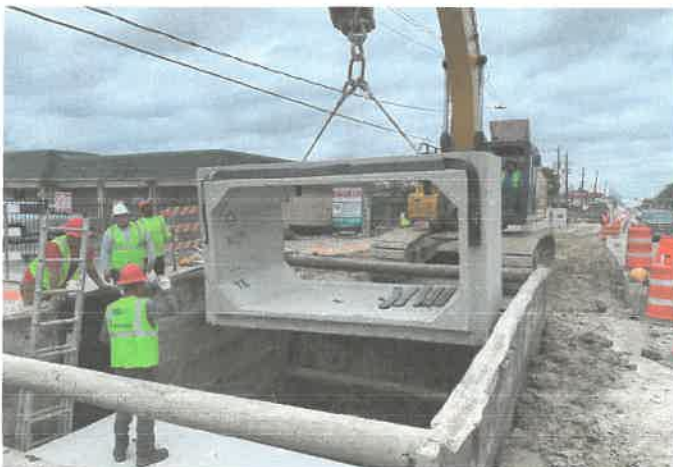
10-FT x 5-FT RCB Installation
