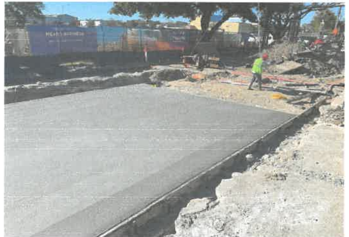
Pavement installation commenced.
