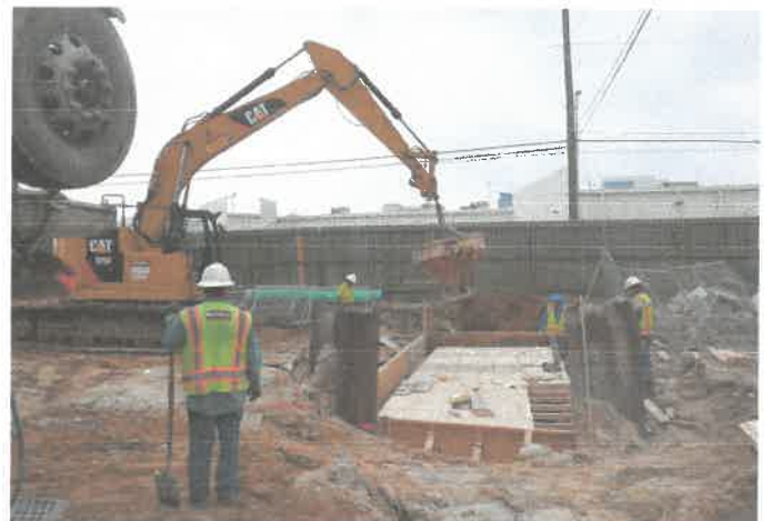
Pouring concrete at Junction Box.
