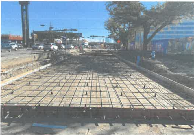
Forming and Rebar for pavement installation.
