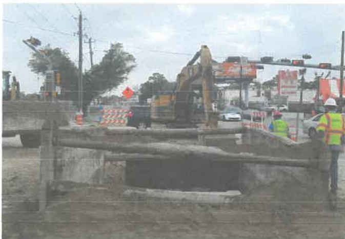
10-FT x 5-FT RCB Installation
