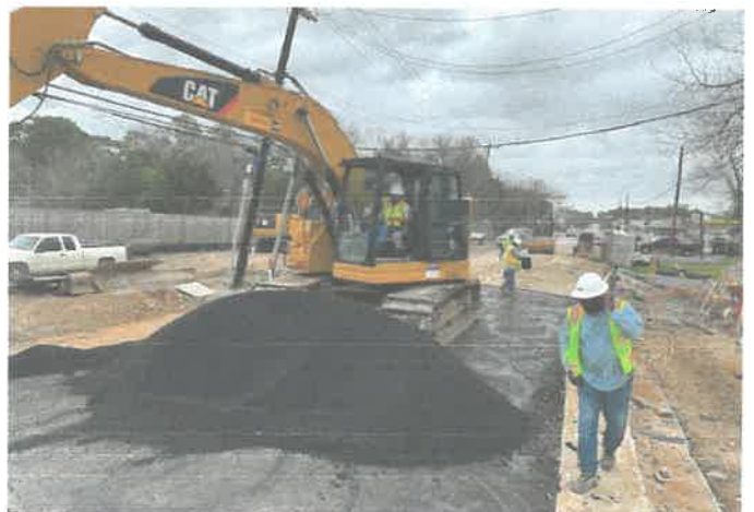
Type D Material being placed
