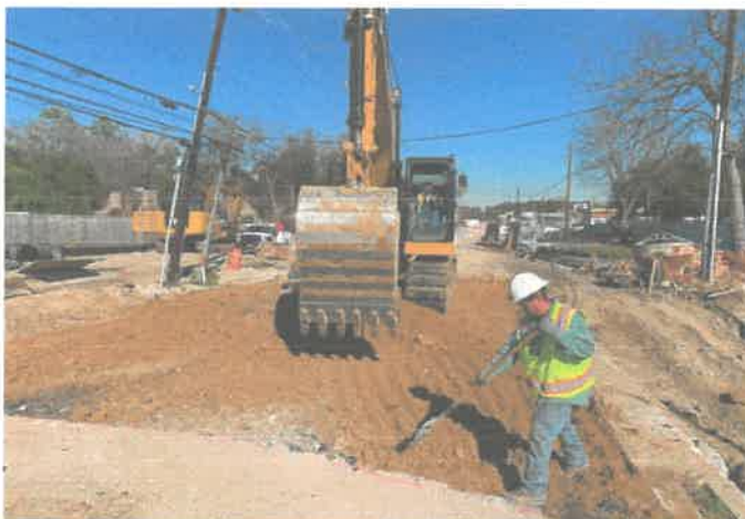
Grading stabilized sand on Witte
