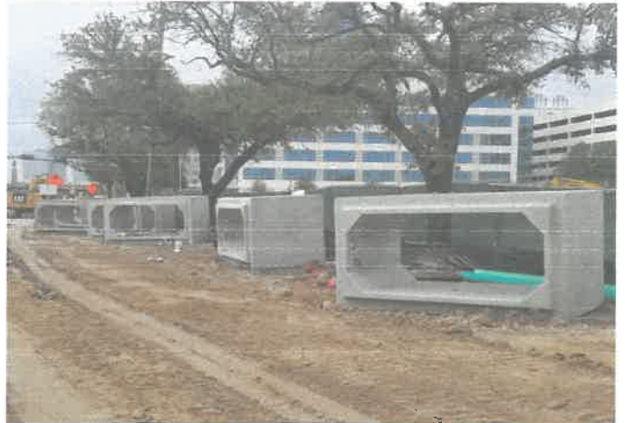
Stockpiled 10-FT x 5-FT RCBs
