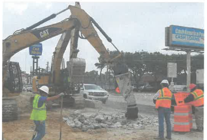
Ongoing Demolition Work
