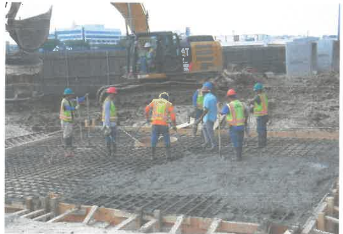
Junction Box Installation
