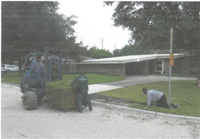
Placing sod on Springrock
