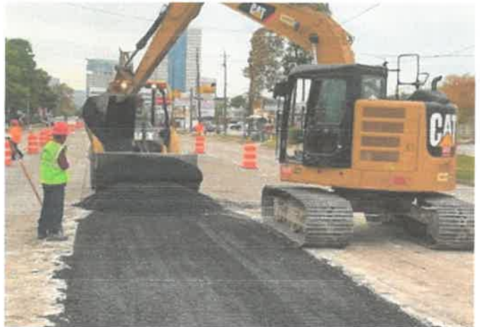
Laying asphalt in medians
