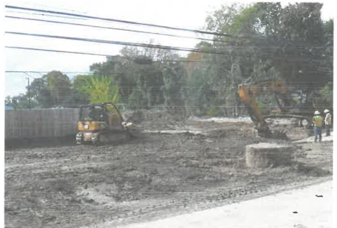
Backfill and cleanup along Witte Rd.
