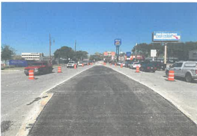
Asphalt installed in medians
