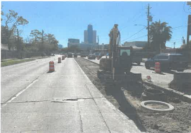
Removal of concrete medians
