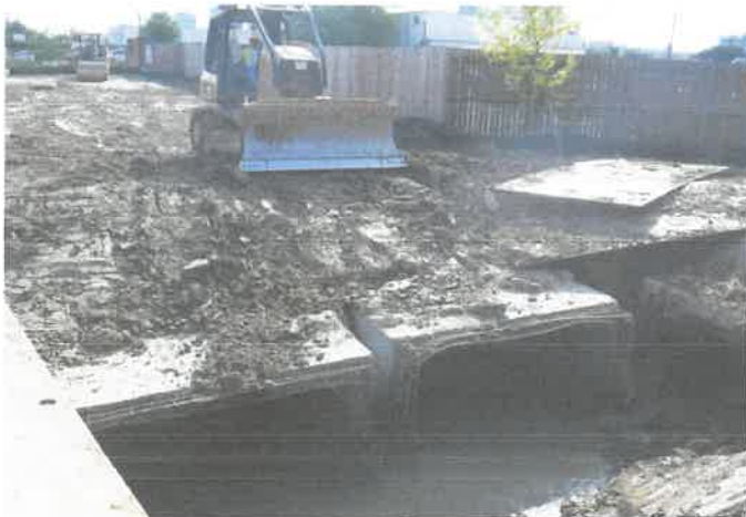
Preparing for junction box installation at Witte Rd.
