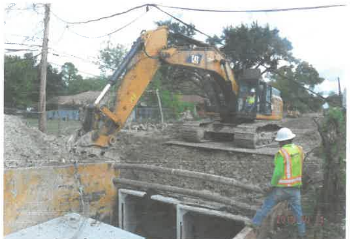
RCB installation under low hanging line — Phase II
