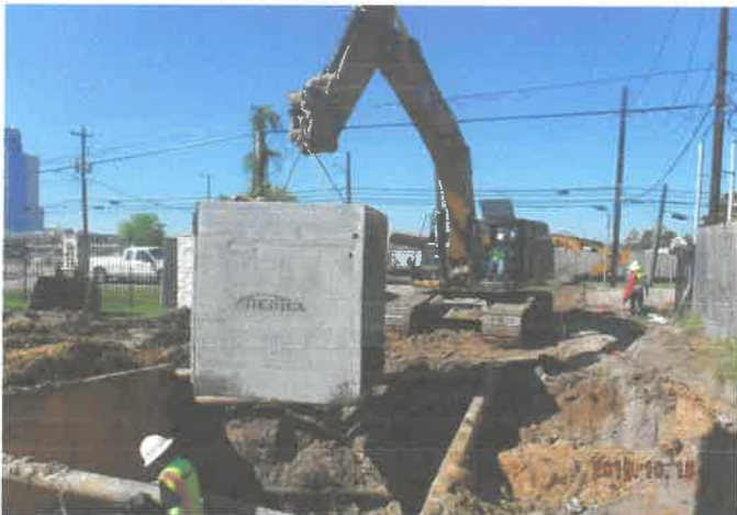
RCB installation — Phase II
