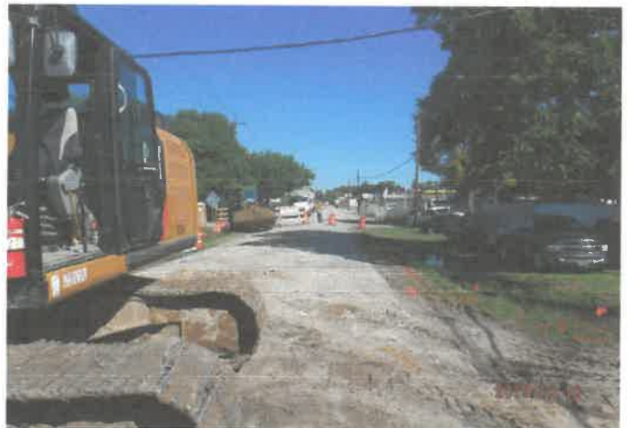
Road closure at Witte Rd in preparation for water line lowering
