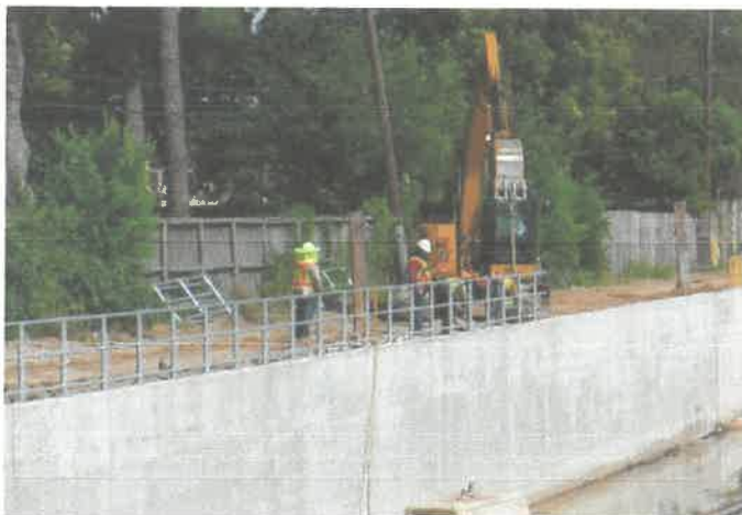
Rail installation on access road — Phase I
