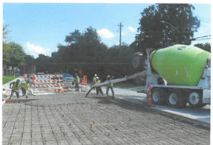
Repaving of Bunker Hill Road
