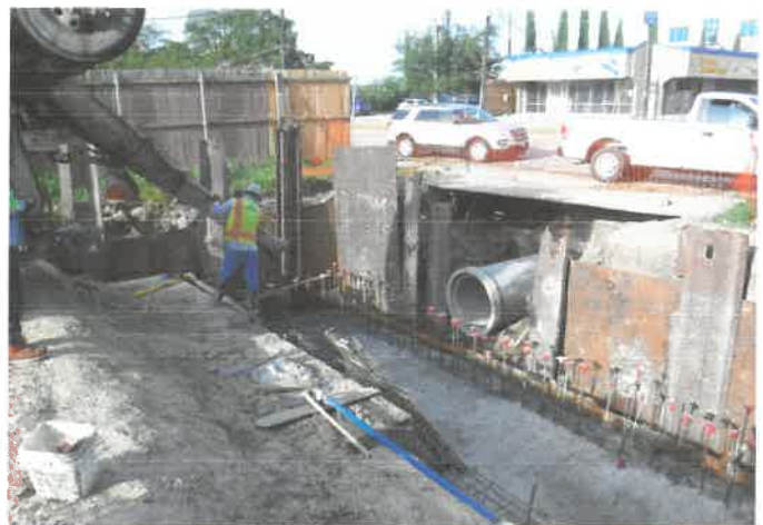
Pouring floor in junction box near Gessner Road
