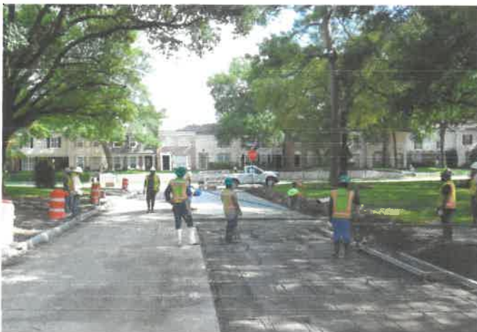
Repaving of Springrock Lane
