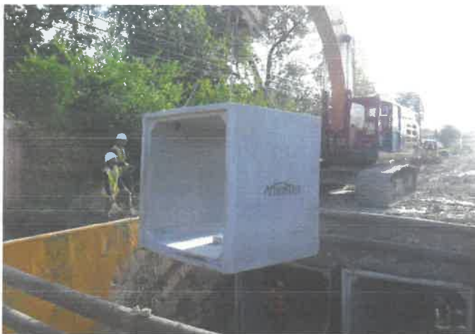
RCB installation west of Bunker Hill Road — Phase II
