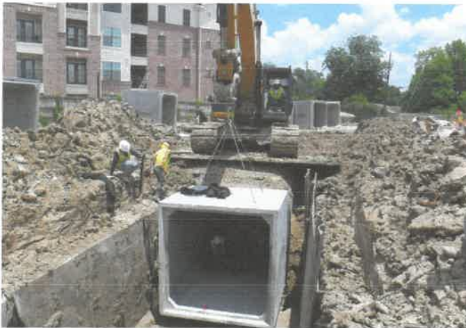
RCB installation west of Bunker Hill — Phase II.
