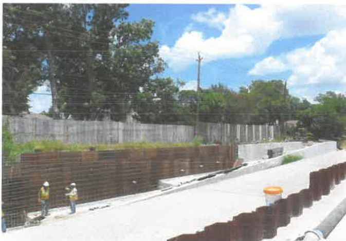
Retaining wall construction.
