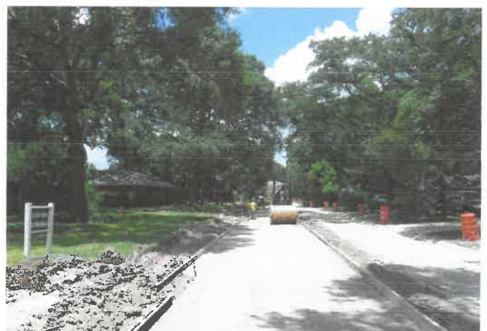
Final compaction before rebar placement on Springrock
