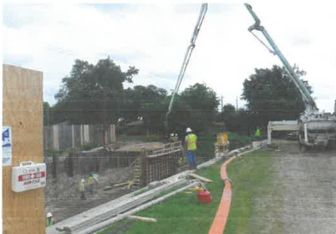
Pump truck used to pour retaining wall.
