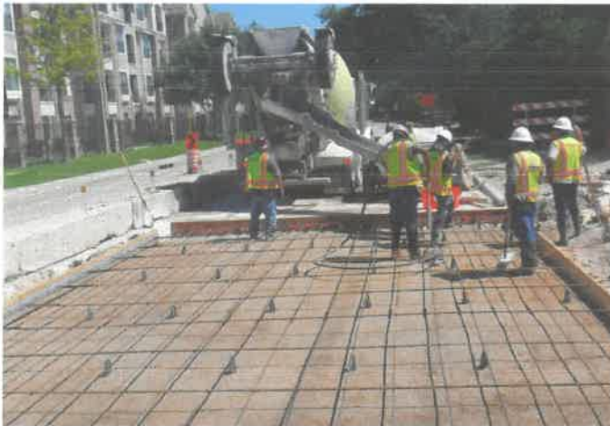
First concrete truck pour on Bunker Hill — east side.
