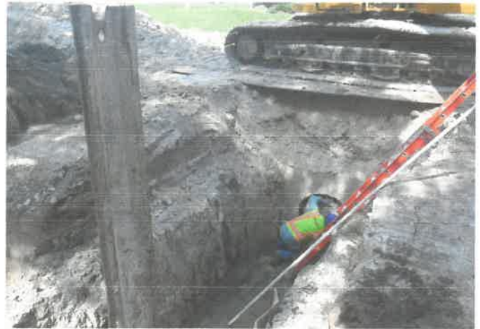
Inlet installation on straw five.
