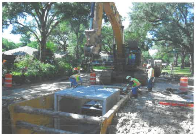
7x7 RCB installation on straw five.
