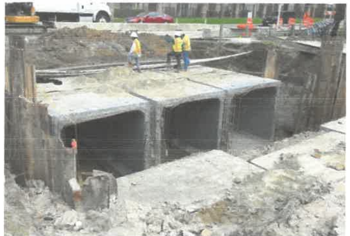
Three rows of RCBs installed at Bunker Hill crossing
