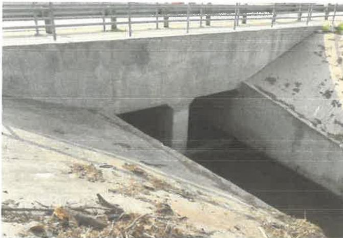
Existing crossing at Bunker Hill looking east cleared from Debris
