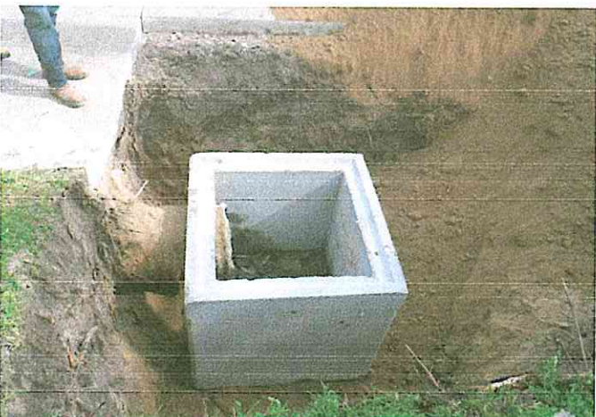
Installation of C-1 inlet along Larston @ Cederdale
