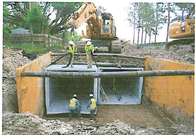
10' x 8' and 9' x 8' RCB Installation—PH I
