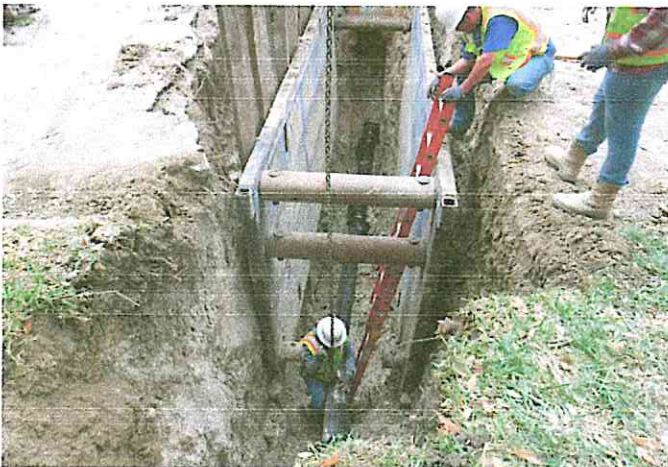
Installation of water line @ Springrock Ln and Pine Lake
