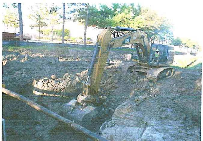
Removal of concrete channel lining
