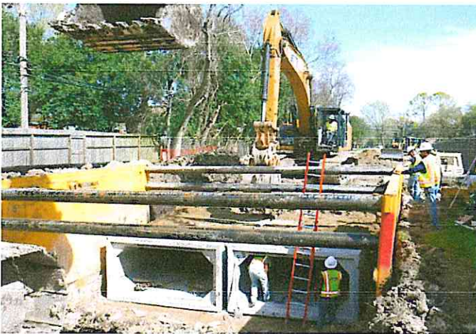
8' x 4' RCB Installation — PH III
