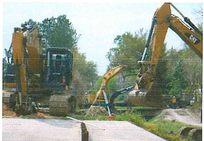
Prep work for 9' x 8' RCB Installation—PH I
