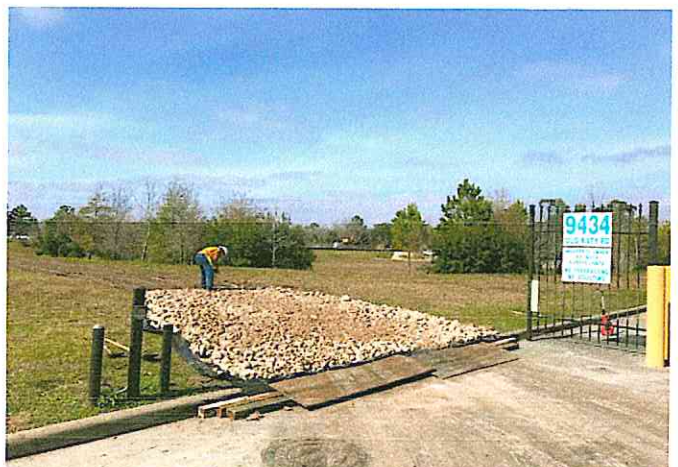
Stabilized Construction Entrance at W140 Detention Basin
