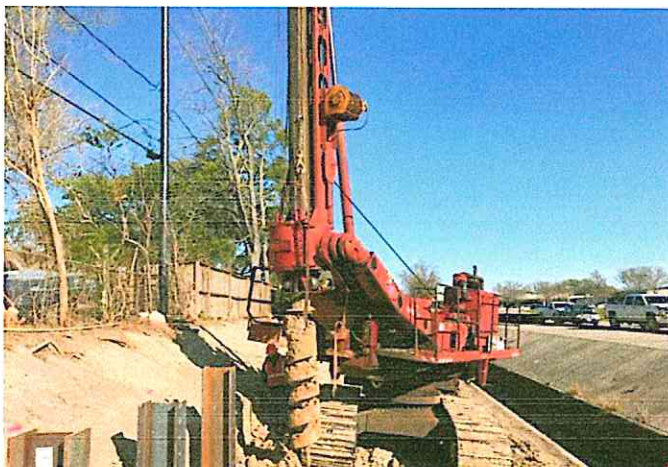
Temporary Shoring Installation
