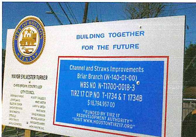
Project Sign Installed
