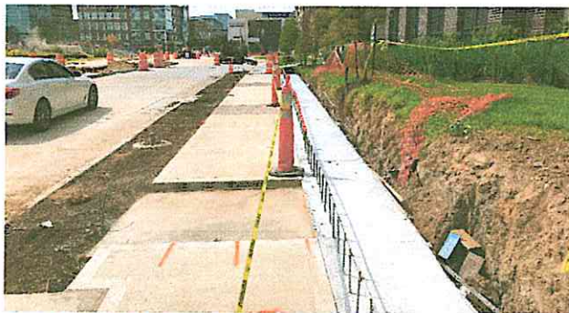
Retaining wall footing at Town & Country Blvd.
