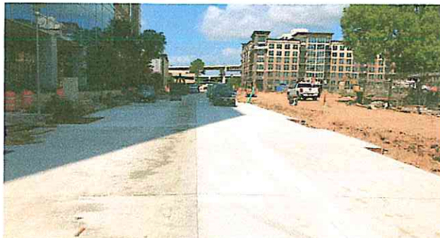
New concrete paving along Town & Country Way—Looking West
