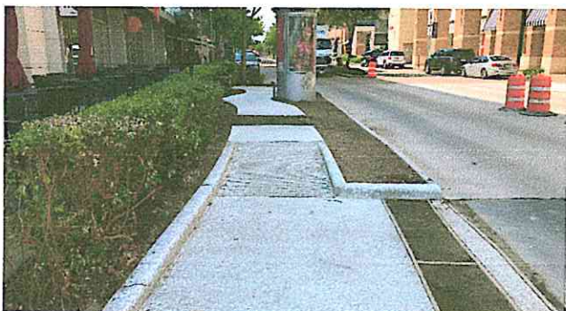
New sidewalk along Town & Country Blvd. in CityCentre
