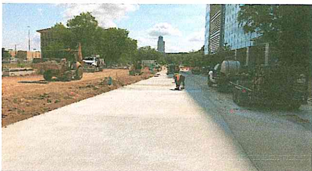
New concrete paving along Town & Country Way—Looking East
