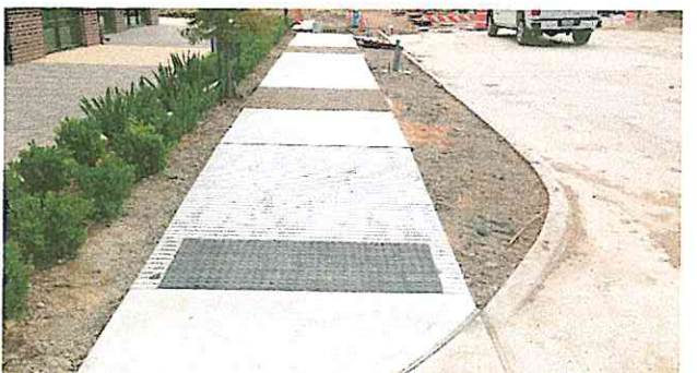
Decorative sidewalk paver inserts installed along Town & Country Way
