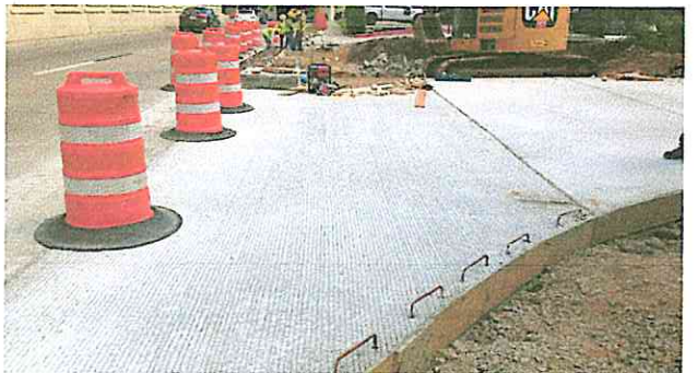
Constructing Town & Country Way connection to BW8 frontage road
