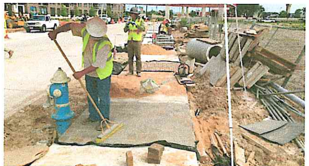
Installing decorative sidewalk paver inserts along Town & Country Blvd.
