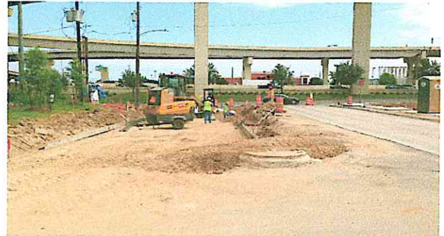
Constructing NB Town & Country Blvd. - looking north
