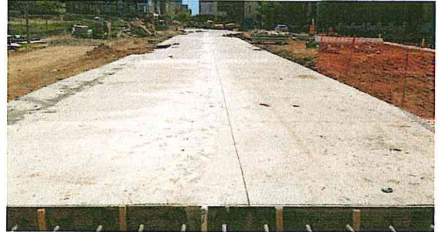
Town & Country Blvd. concrete pavement in progress—looking south
