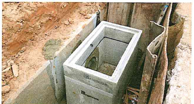
New storm water curb inlet bottom section
