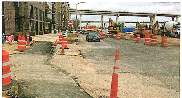
Work continues along Town & Country Blvd. (looking north)
