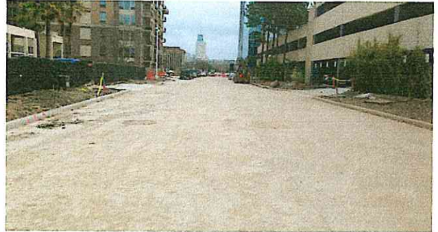
Town & Country Way extension looking east
