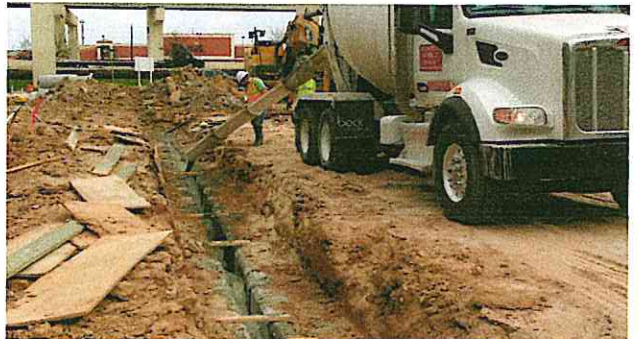
Placing flowable fill between storm water box culverts
