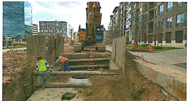
Installing storm water detention boxes along Town & Country Blvd.
