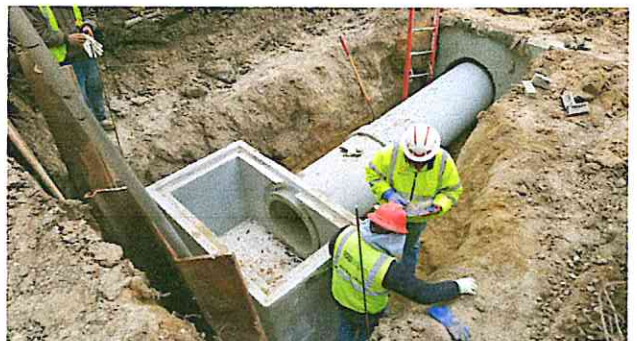
Installing storm sewer inlet
